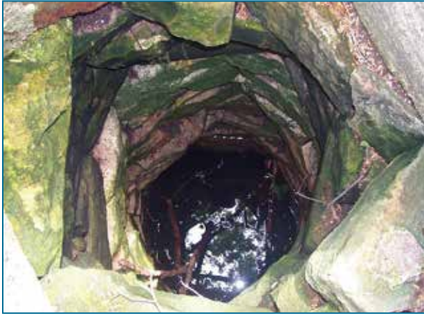
FIGURE 62. Improperly unplugged, abandoned wells can be a source of groundwater contamination.
