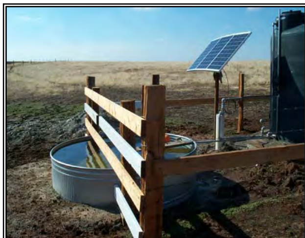
Figure 7 – PV solar array with storage tank and stock. (Source: “Renewable Energy Primer-Solar.”)
