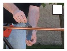
**Step 1**Before installing the Add-A-Valve®, clean the copper tubing with a fine emery cloth to a bright shiny finish.
