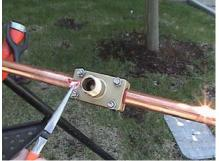
Note: To flush debris, reverse the stem cutter with bottom cap off until you see a flow of water. Debris should be flushed. Reseat the valve until the flow stops and replace cap. Congratulations, shut down is now complete! You can now use the Add-A-Valve® to make a repair or as a live, hot tap. The Jomar Add-A-Valve® is engineered for ONE-TIME use as an emergency shut-off device! Once the stem cutter has been raised DO NOT lower it again.
