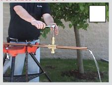
Use a 3/8" socket wrench, manual operation only! Do NOT use a drill motor.
