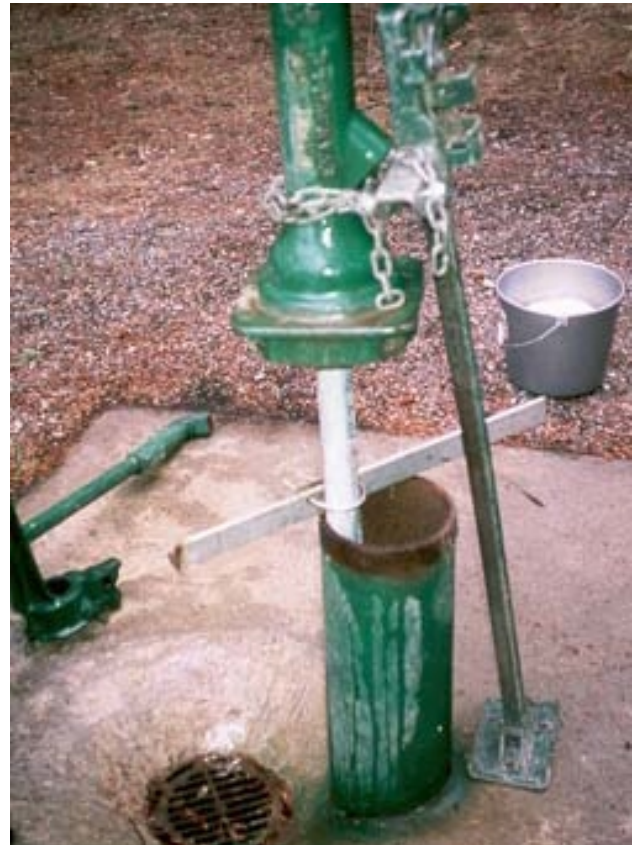
Figure 18—U-bolt attachment of the steel angle to the drop pipe.
