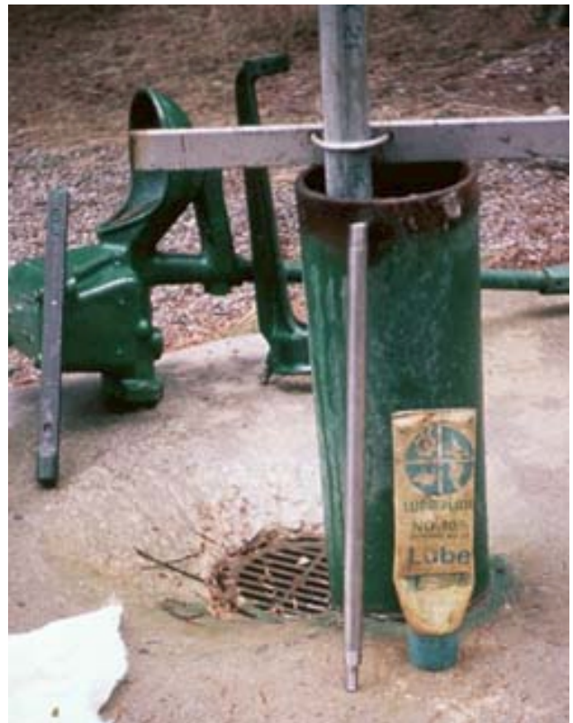
Figure 21—LUBRIPLATE No. 105 is used to lubricate the pump during reassembly.
