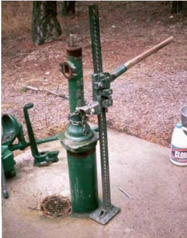
Figure 16—Attachment of the jack to the pump base.
