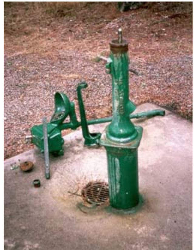
Figure 15—View of pump after removal of the pump cap, upper guide, flat piston bar, packing, packing nut and fountain/reservoir assembly.
