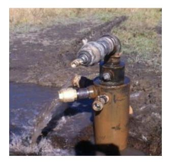
Grout can be pumped from 10+ psi to 70 psi (safety factor) to fill voids between the production casing and the ground formations and to seal the annulus between the production casing and surface casing. The rate at which an artesian formation will accept grout will vary due to the available porosity of the geological unit. For example, coarse, clean gravels will accept pumped fluids at a faster rate than fine grained sand because of the pore capacity.
