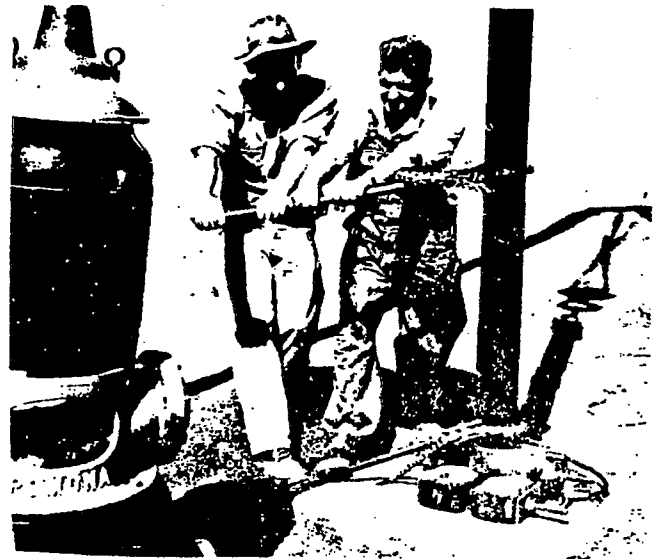
Ill. 18 - Showing proper method of tightening column coupling. By properly attaching chain tongs, the column pipe will not be dented or damaged.
