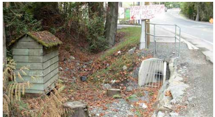
FIGURE 9 Dug well (in well house) near culvert & busy road
