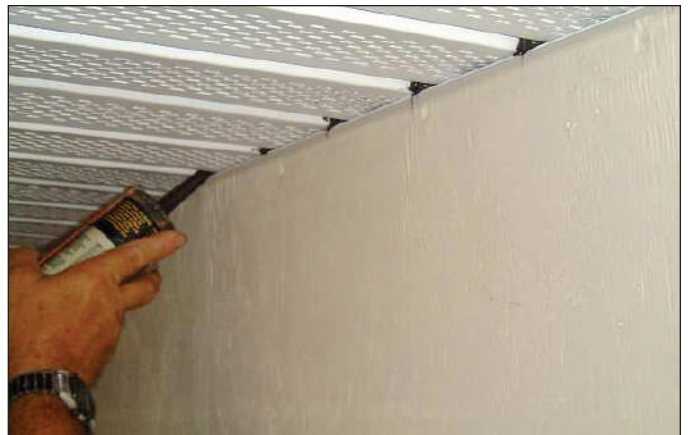
Figure 4. Applying dabs of sealant.
