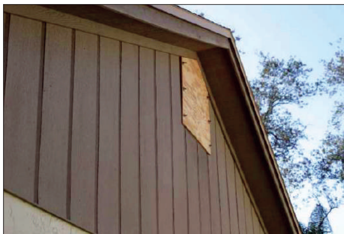
Figure 10. Shuttered gable end vent.
