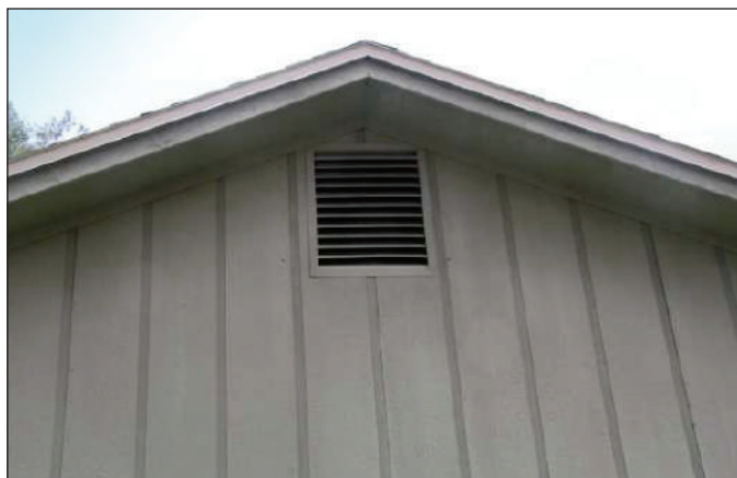
Figure 9. Gable end vent.
