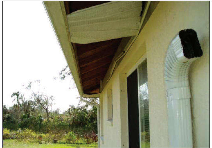
Figure 1. Missing soffit material.
