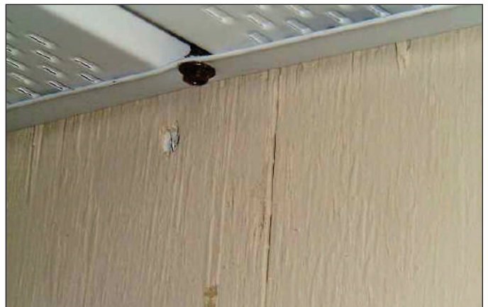
Figure 5. Screws through wall channel.
