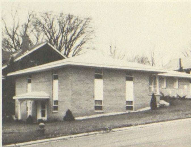
Figure 27. A house planned and constructed for cold-roof performance, but without the expense of the double roof structure.
