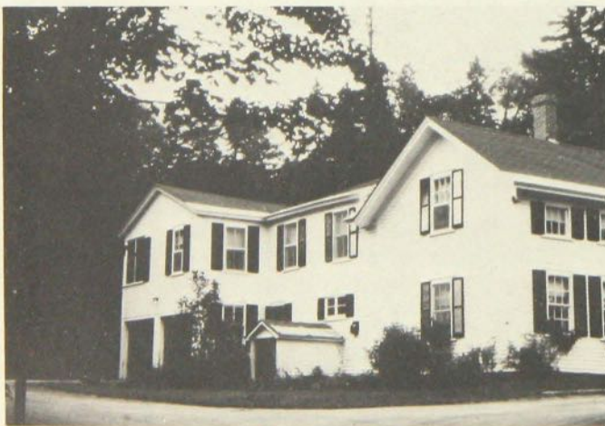
Figure 9. Eave flashings of aluminum.
