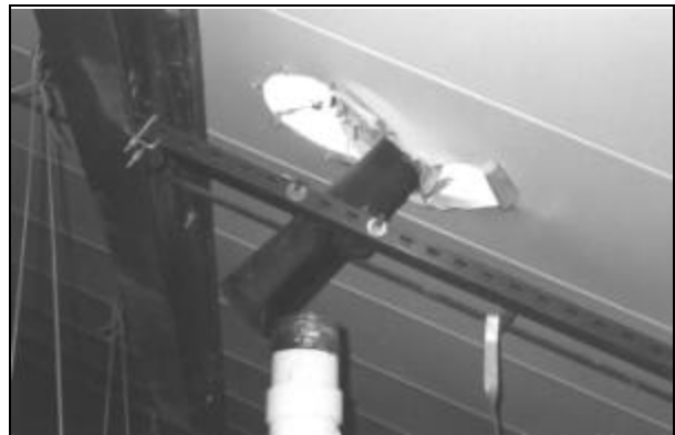
Figure 9. Tear in metal roof caused by plumbing vent displacement shown in Fig. 8.
