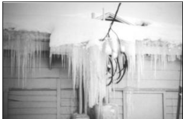
Figure 10. Electrical service entrance cables should not be located below cold eaves.
