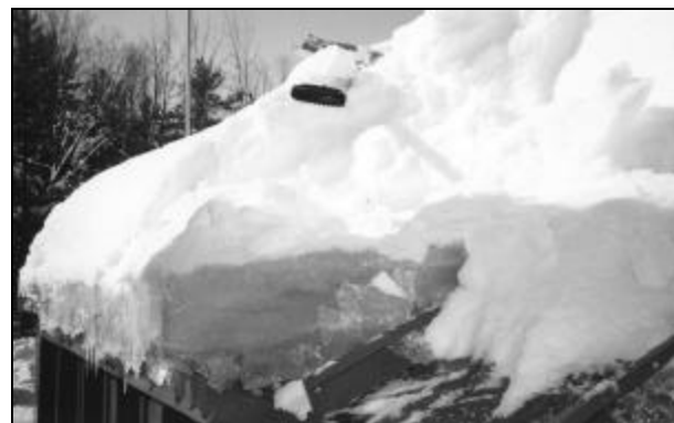
Figure 2. This large ice dam caused this metal roof to leak at its eaves.
