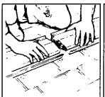
6. Join CRV Ridge Vent sections with connector plugs.
