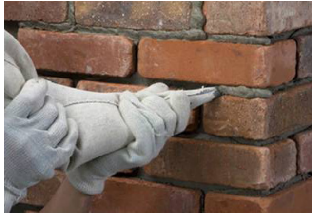
Photo 2 Mortar Placement Using a Grout Bag
