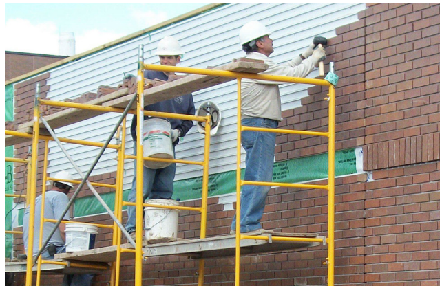
Photo 3 Installation of Modular Panel
