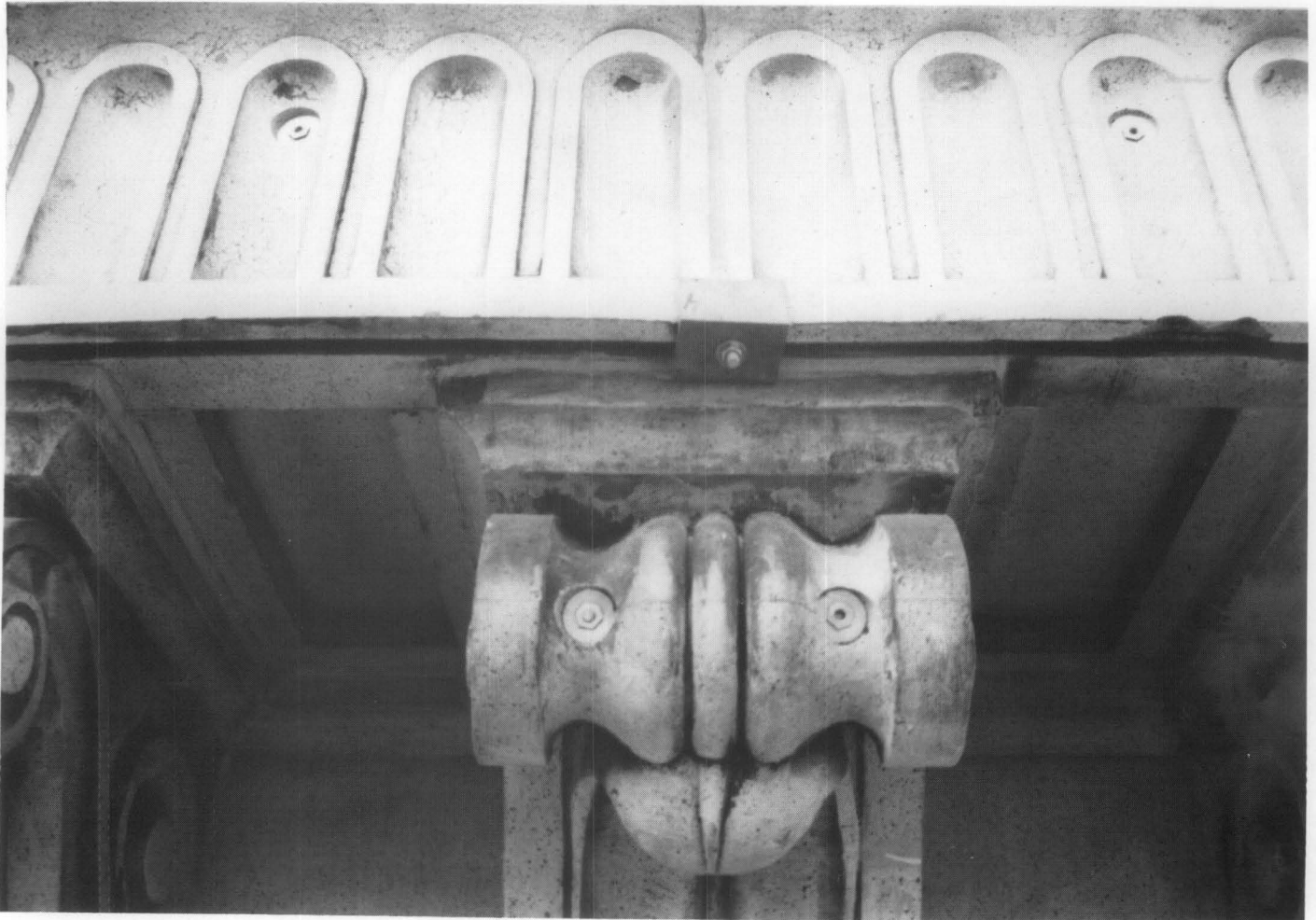
Figure 11. Completed anchor installations at a fascia and bracket. The countersink holes penetrate no more than half the thickness of the outer wall of the terra cotta and were filled later with epoxy.
