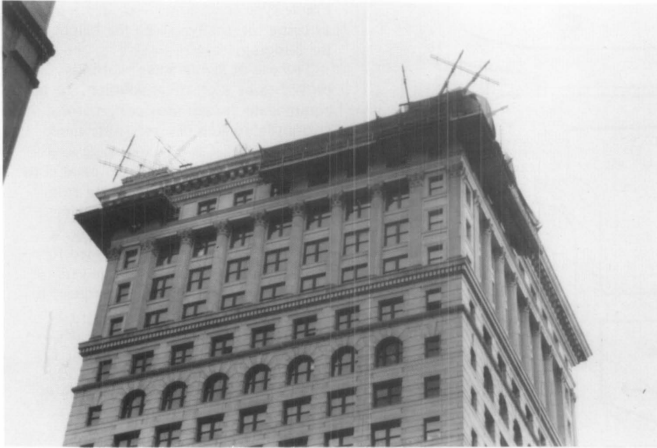
Figure 8. Access to the cornice was provided by cantilevered aerial scaffolds at the southeast and southwest corners of the cornice. All other locations were accessed by hanging two swing stages, side by side. The inner swing was hung off of a V-shaped bracket (shown) while the outer swing was hung from a steel deadman which projected horizontally across the cornice roof. Both the V-shaped bracket and the deadman were designed to transfer the weight of the swings vertically down through the center of the cornice. No load was placed on the outer edge of the cornice. Photos by Jeffrey S. Levine.
