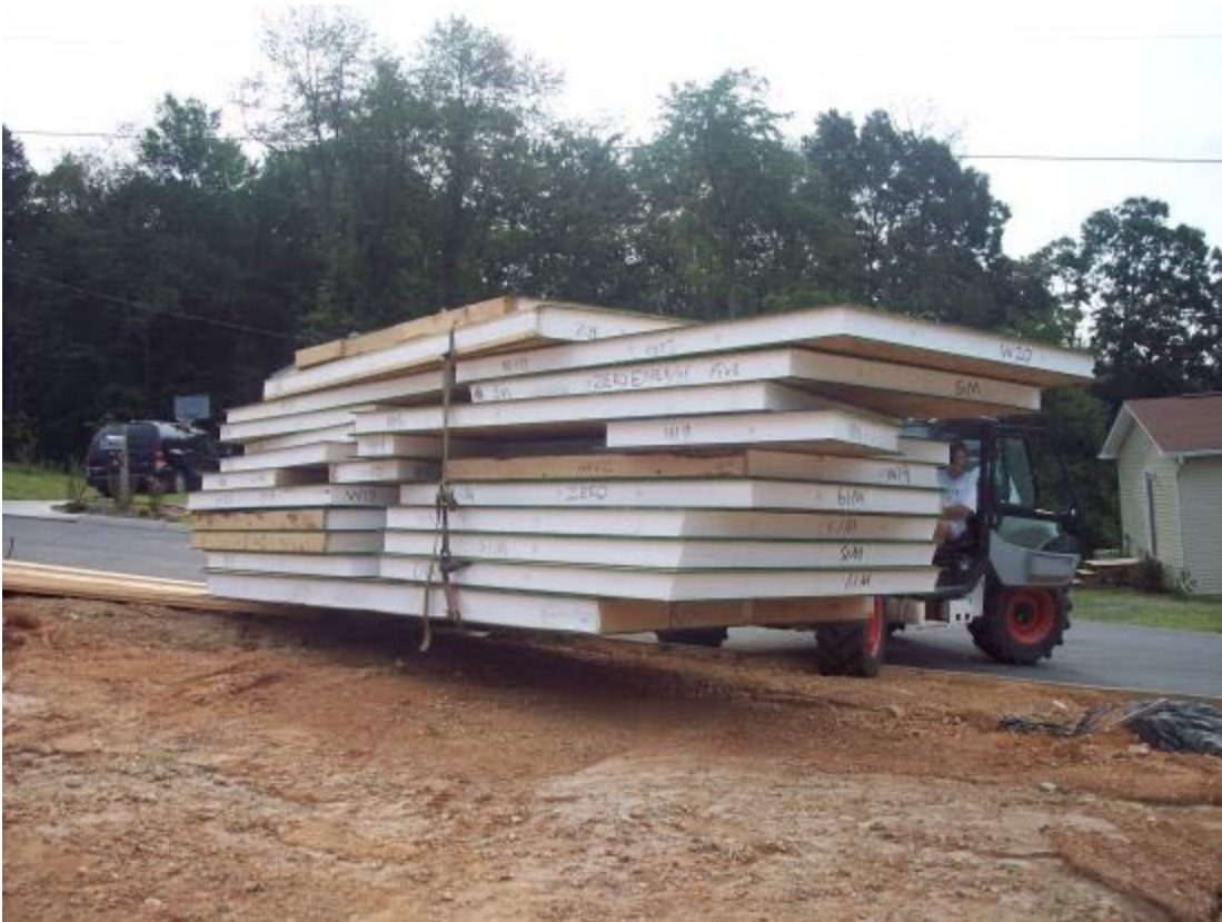
Figure 3. An all-terrain forklift is used to move and stage the panels.
