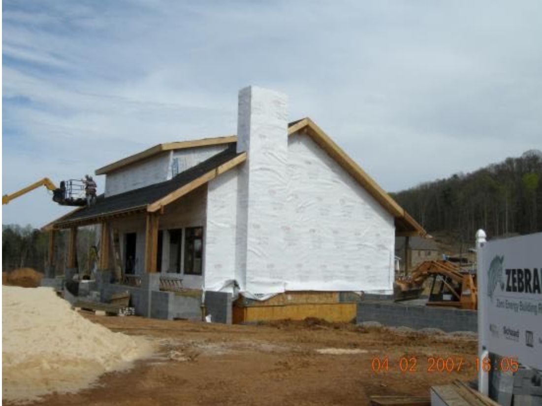
Figure 15. Two layers of high-permeability house wrap are installed to provide a drainage layer between the SIPs and the homes external cladding.
