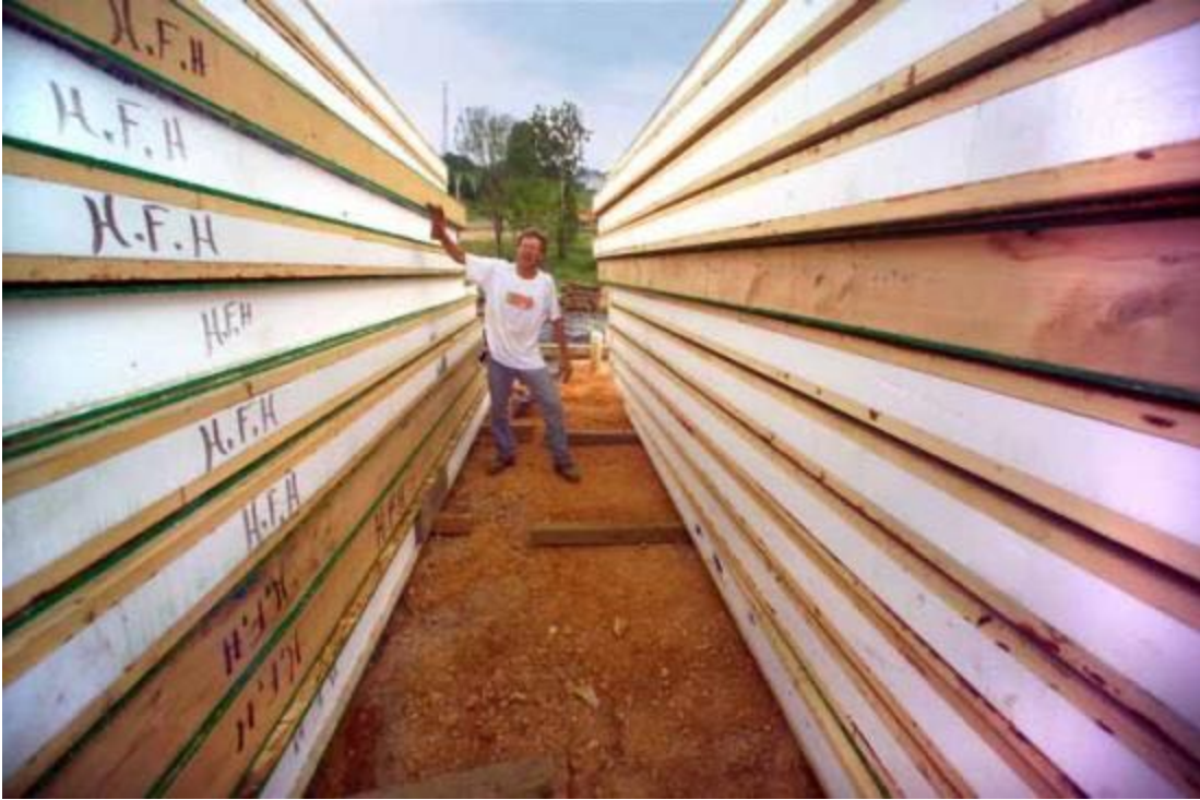
Figure 2. SIP panels should be stacked high, dry, and flat.
