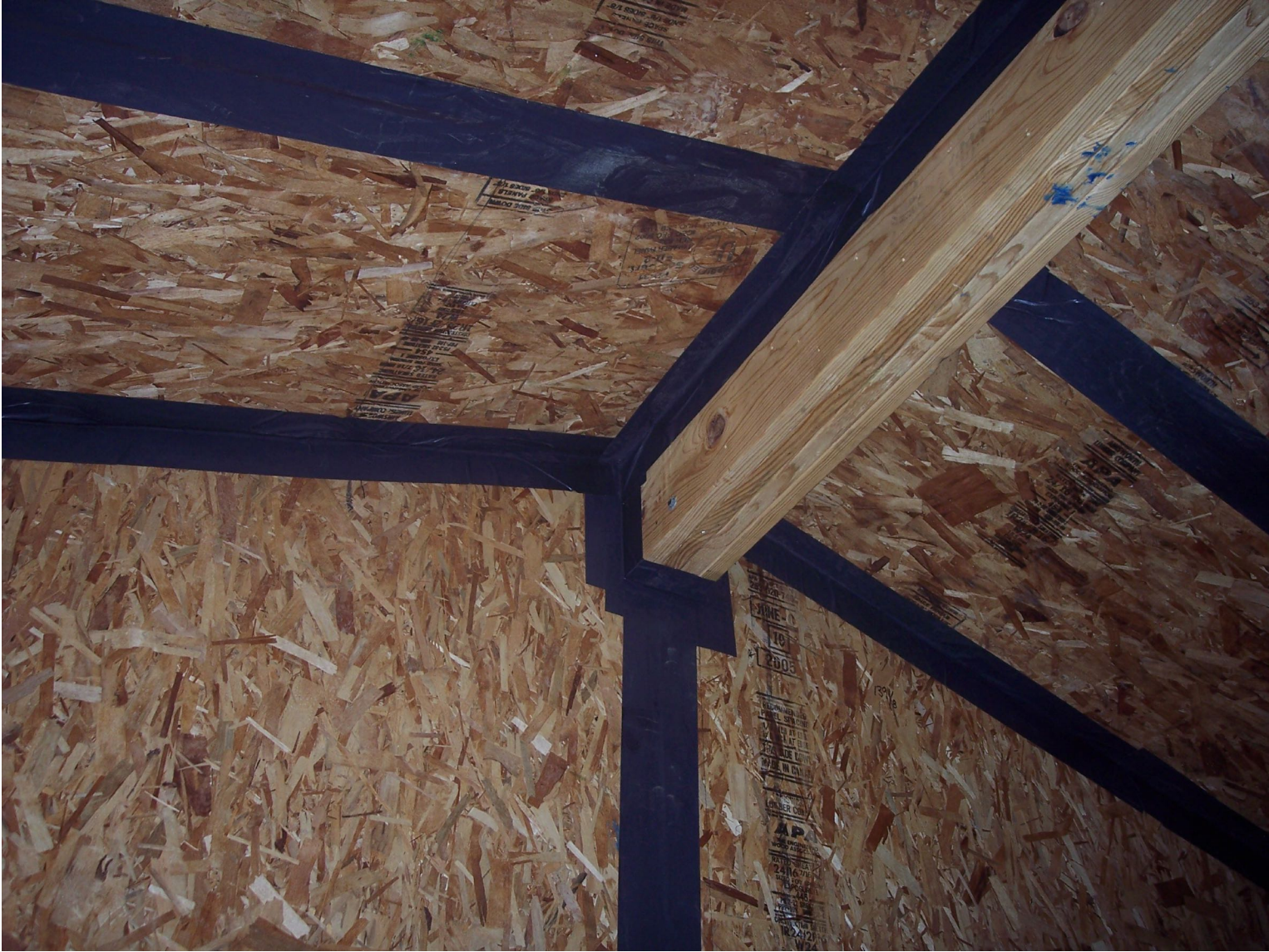
Figure 12. Peel-and-stick panel tape provides added assurance that SIP panel seams will remain airtight (Source: ORNL (http://basc.pnnl.gov/library/ornl/) ).
