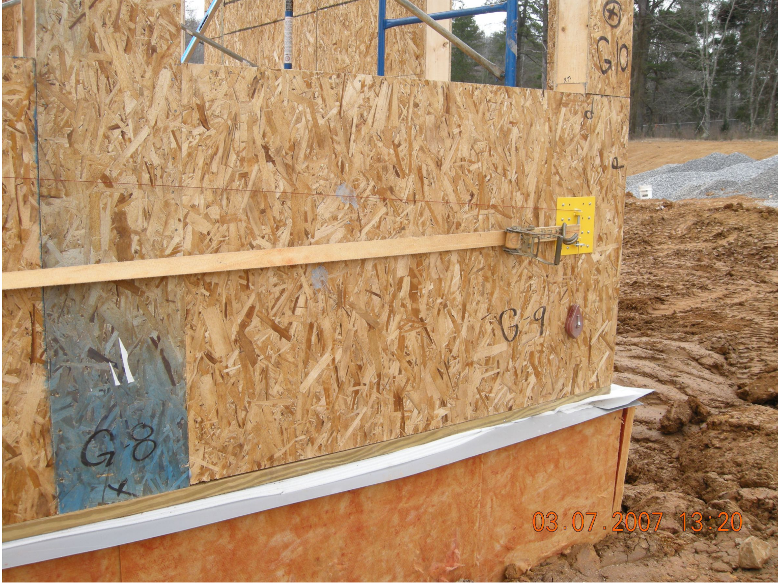
Figure 11. Lifting plates attached to the wall provide good bracing to tighten up SIP panel seams (Source: ORNL (https://basc.pnl.gov/library/ornl/) ).
