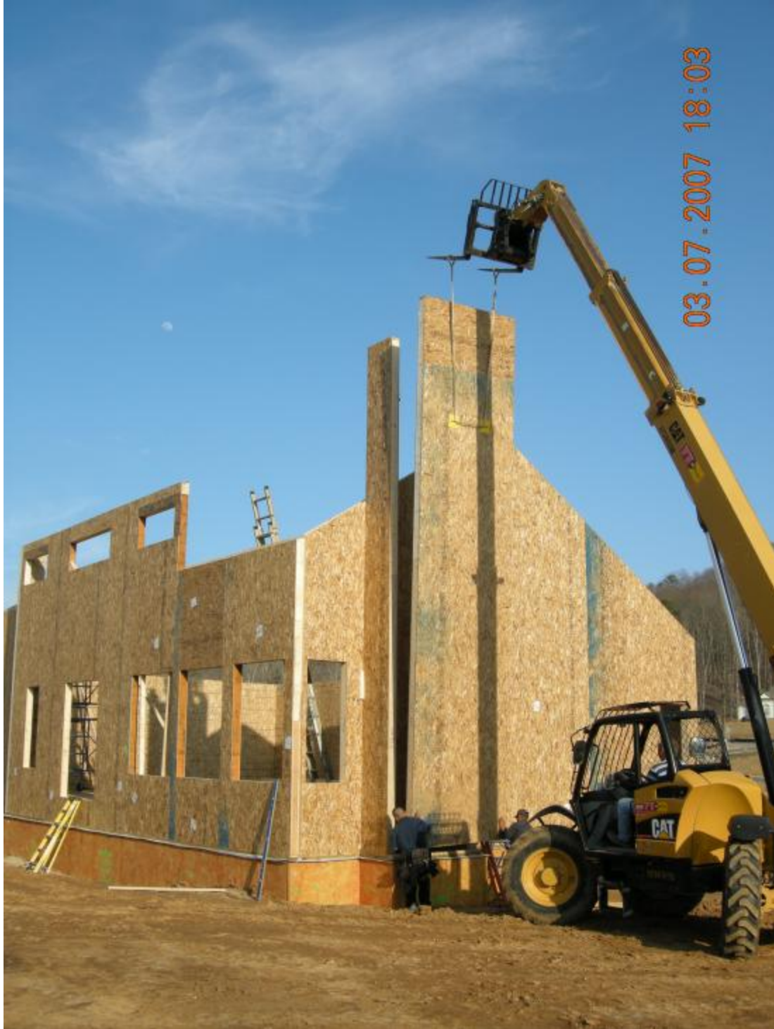
Figure 6. A crane is used to install the SIP fireplace chimney chase.
