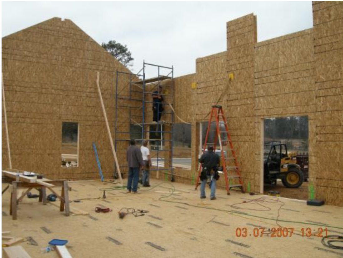
Figure 5. Walls are being assembled at this SIP house.
