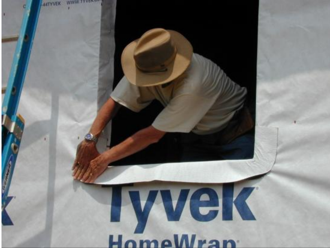
Figure 16. After installing the house wrap over the SIPS, window flashing is installed (Source: BSC 2009 ( https://basc.pnnl.gov/library/builders-guide-structural-insulated-panels-sips-all-climates )).
