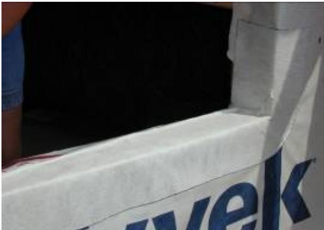
Figure 17. The back dam of the window sill will force water out.
