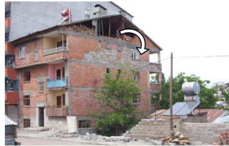
(b) Falling of gable wall caused death of a child
