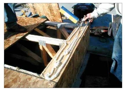
Proper sealing is especially important when installing SIP roofs. The ridge of a SIP roof can use either bevel-cut SIPs for a flush joint, or use a beveled foam block insert. The ridge detail is a critical construction detail that requires attention to sealing using methods as noted above. Manufacturer specifications will provide specific sealing details designed to prevent moisture movement.
