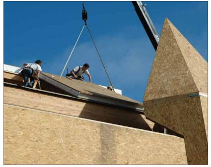
SIPs are often cut using optimization software that minimizes the amount of waste. EPS waste generated in the SIP manufacturing and fabricating process is recycled into other EPS products. Jobsite waste is also reduced.
