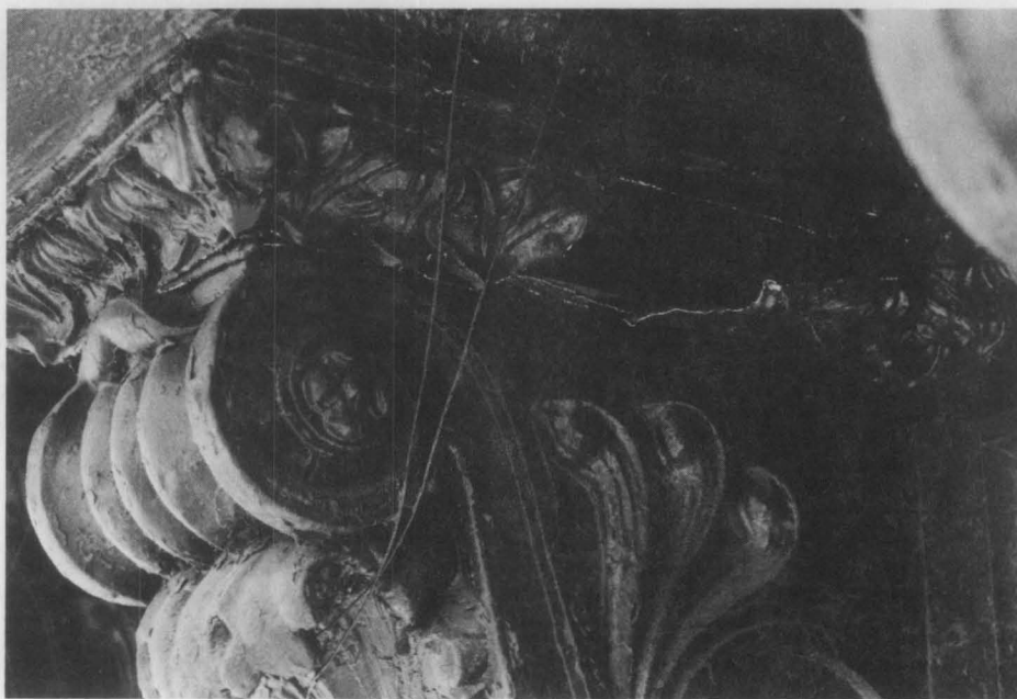
Figure 4. As shown in this view, the molding applied to the modillions was extremely deteriorated. A more serious problem was that most of the zinc modillions had fractured where the integral leaf moldings met the scrolled sides, allowing them to separate from the soffit. As a previous temporary safety measure, holes had been cut in the soffit panels to pass supporting wire beneath the modillions. Photo: Richard Pieper.
