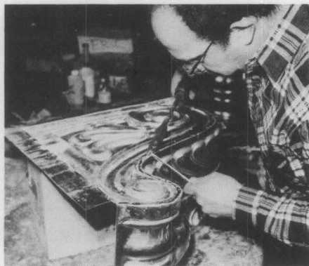
Figure 8. The modillions consisted of 6 stamped pieces soldered together by the installer. Photo: Richard Pieper.
