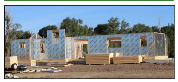
RAYCORE Structural Insulated Wall Panels are not meant to be a finished and exposed surface. Internal surfaces of panels should be covered with a minimum 15-minute thermal barrier, such as 1/2" gypsum wallboard or other approved materials. External surfaces of panels should be finished as soon as possible with materials that provide protection from sunlight, weather, moisture and all elements.
