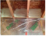
reducing it's effectiveness. Although spray foam is not a great insulation choice, it is a very good air sealer. Consider adding 2" to 6" of spray foam to each floor's rim board and back it with and additional insulation whether it be fiberglass, cellulose, rockwool or even panel scraps to achieve at least an R-value equal to that of your walls.
