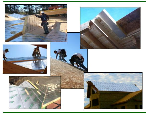
RAYCORE Structural Insulated Panels used on the roof should be fully protected from sunlight, moisture and the elements utilizing tarps, roofing materials or other means to provide temporary protection and permanent roofing materials should be applied as soon as possible upon the completion of installation. The panels are not meant to be left as a finished product.
