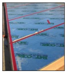
To get the best performance and ensure that there be no air infiltration and resulting vapor transference, all seams, joints to additional framing members, and penetrations should be sealed with vapor proof tape. (FSK tape can be supplied by RAYCORE.)
