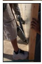
Apply a continuous bead of foam friendly construction adhesive to the bottom plate to provide an airtight seal to subfloor and stand wall.
