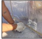
bottom plate at the anchor bolt locations. Number and reserve the foam blocks as they will be reinserted, filling the voids once the bolts are secured to the bottom plate. Predrill bottom plate for bolts.
