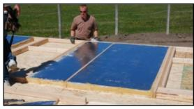
frame your first corner. Start laying panels out, cutting panels when necessary. When your wall meets a door or window simply cut the panel so it butts tight against the king stud on the window or door frame, and use cut material to continue on the side opposite the opening, cutting where
