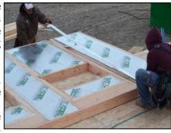
to additional framing members, and penetrations should be sealed with vapor proof tape. (FSK tape can be supplied by RAYCORE). Although care should be taken to prevent damage of the panels and their foil facing when handled, small tears, occasional bumps or gouges may occur. The panels can be simply repaired by filling with canned polyurethane foam or by applying vapor proof tape.
