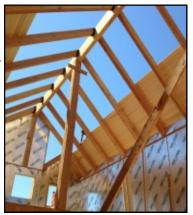
**Best Practices:** Spread 6 mil visqueen, roofing felt or other vapor barrier over entire roof decking surface under panel. If no decking is specified, underside of panels should be taped with 3" vapor proof tape, and all joints check and filled for a tight seal, to prevent air infiltration or moisture transfer.
