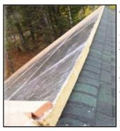
Adding Insulation To An Existing Roof: RAYCORE's lightweight, easy to use, modular roof panels with integrated framing member or "studs" is the perfect solution for adding insulation to the roof of an existing structure without disturbing the interior of the home. Simply frame the edge of the roof extending fascia and soffits and apply panels to existing roof. Deck as required, and apply roofing in an appropriate manner.
