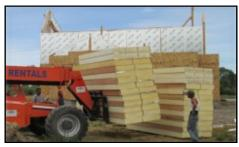
It is advised that when possible, a forklift with fork extensions and an operator be available. If this is not possible, the panels can be
