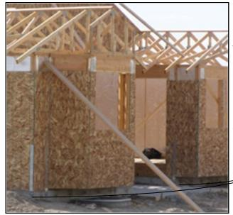
Hurricane Straps example (ie. Simpson STHD straps). As you would with conventional stick framing, hurricane straps are nailed into the RAYCORE Wall Panel's integrated studs. If the integrated stud in the panel does not line up with the STHD strap then you will need to place a stud in proper location during the framing process.
