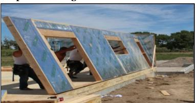
Sheathing can be attached either before or after the wall has been raised. Framer's preference.
