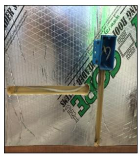
Once inspections have been performed and rough wiring has been approved, backfill channels and penetrations with canned polyurethane foam (Great Stuff or equal) and once cured, remove any excess.
