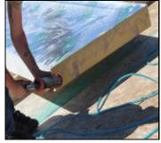
To ensure an air-tight joint, apply a continuous bead of foam friendly construction adhesive, (such as Liquid Nails or equal) to all edges, between the panels and all other framing members to seal joints. Push panels firmly together, leaving no gaps and assuring the panels are tight and square. Attach to roof as instructed in Step 3. Further sealing, if required, can be performed once the panels are permanently attached.
