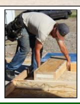
**Step 2. Wall Layout:** Establish your layout by starting with your corner (See Step 3 & 4), placing lumber, measuring and marking top and bottom plates, and laying out panels, door and window frames, etc.
