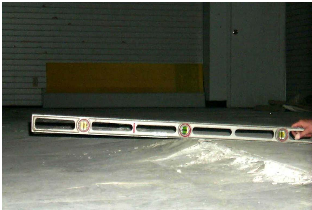
Figure 3.15 – Vertical displacement of floor from pyrite oxidation, from (Carter 2002b).
