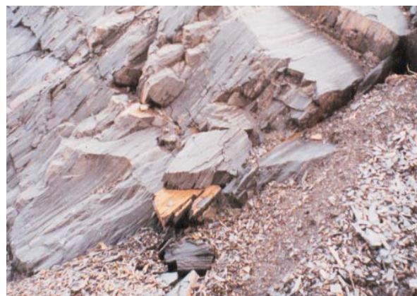
Figure E.8 - Visible evidence of weathering by pyrite oxidation of exposed face of Millboro Shale, along Rte. 100, VA.
