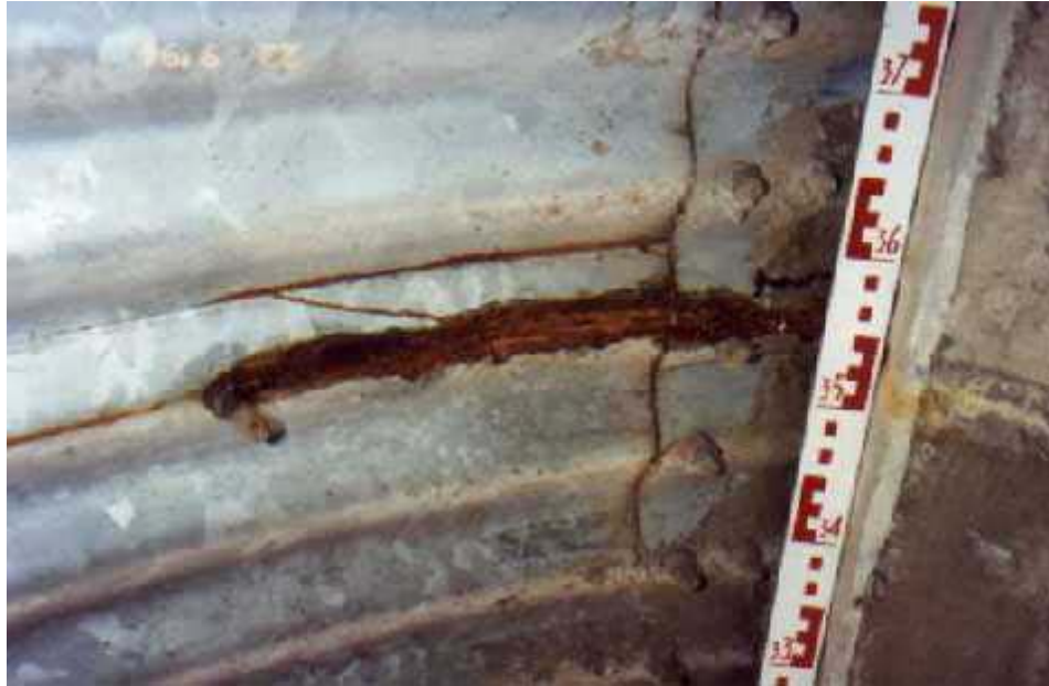
Figure 3.12 – Corrosion of corrugated steel buried culvert from pyrite oxidation. Photo from www.shef.ac.uk/civil/research/gge/ .
