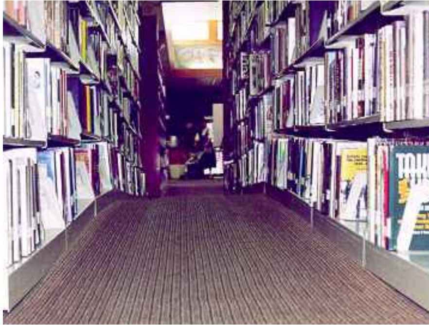
Figure 2.1 – Sulfide-induced heave of library floor and bookshelves at Johnson City Public Library, Johnson City, Tennessee.
