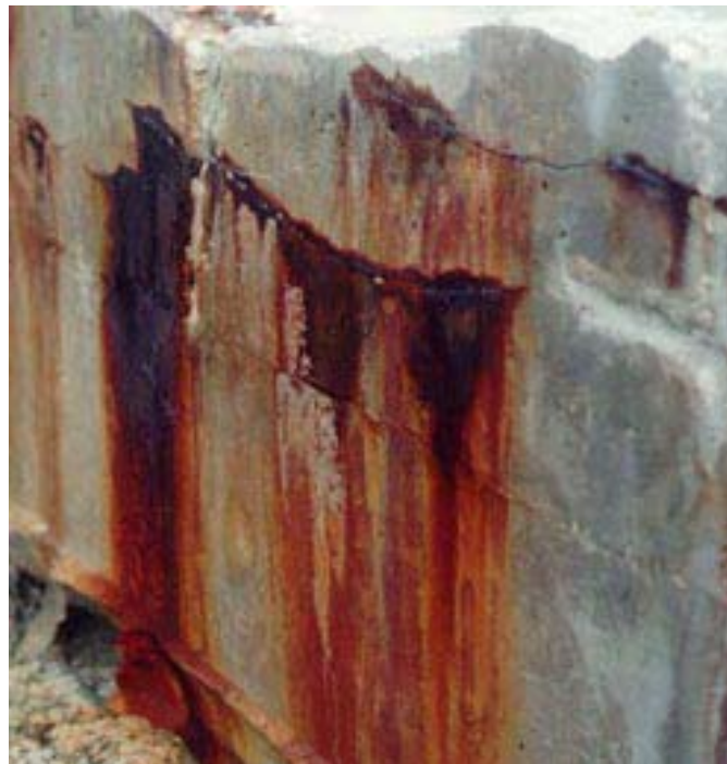
Figure 3.13 – Concrete degradation resulting from “sulfate attack” and corrosion. Photo from http://corrosion.ksc.nasa.gov/ .
