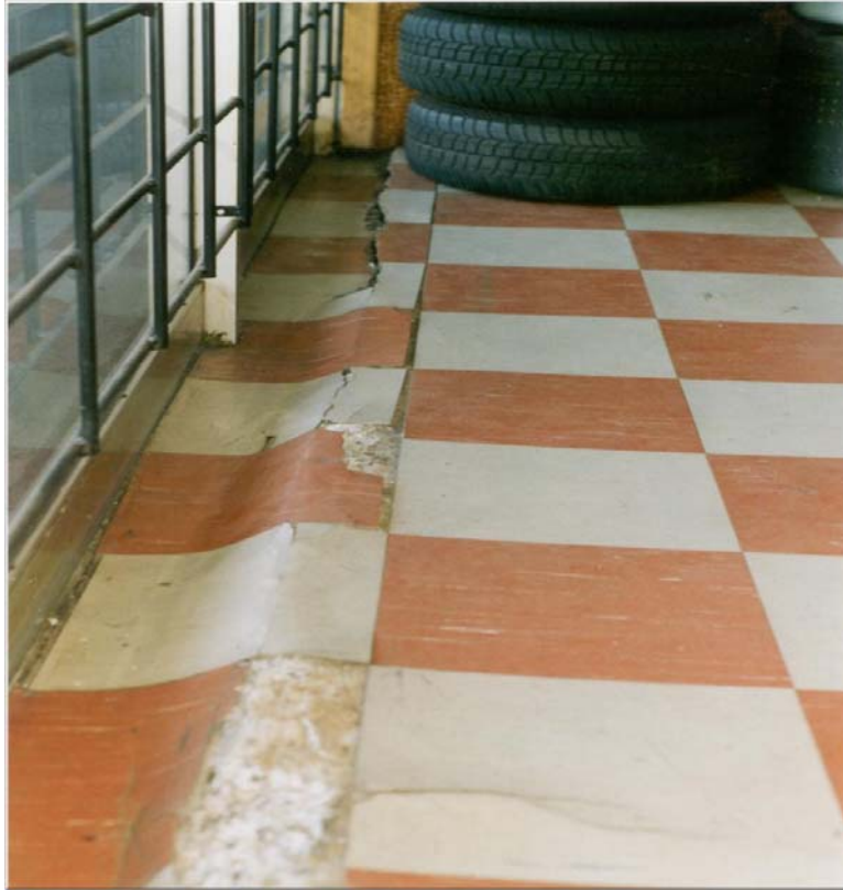
Figure 3.14 – Floor heave resulting from pyrite oxidation, from (Carter 2002b).
