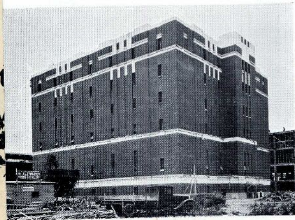
A quarter-million square feet of Fir-Tex is used for roof insulation in this warehouse of Joseph E. Seagram & Sons, Inc., Louisville, Ky.
