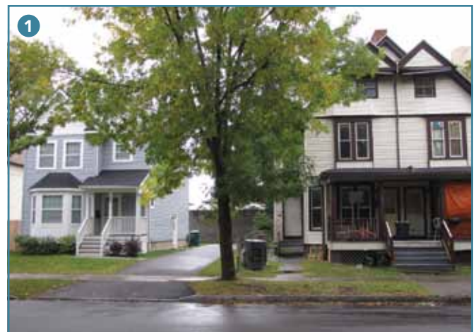
(1) The two structures: 12 Washington Avenue is on the left; 10 Washington Avenue is on right. (Photos by author unless otherwise noted.)
