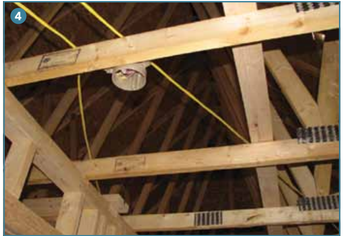
(3) The wood trusses in the attic are 24 inches on center and use gusset plates. (4) Cardboard is used to maintain an opening between attic trusses from the vented soffits for air movement.
