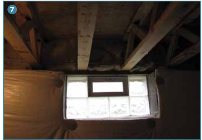
(7) The basement window can be effective for applying water from a hose stream from the exterior into the basement and trusses or I-beams. (8) The tip of the gooseneck applicator is removed, and the water stream has reach and penetration.
