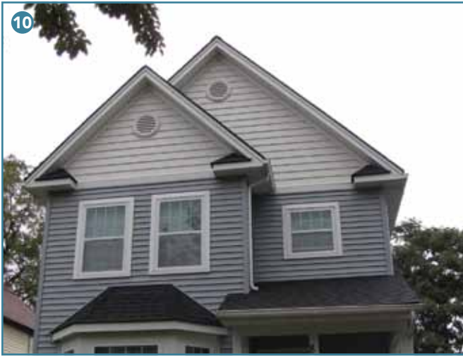
(10) The gable could be an effective way to apply water into an attic fire from the exterior. From a ground or an aerial ladder, use a hand tool to cut a hole from the exterior below the gable and just above the top floor to direct a stream into the attic.
