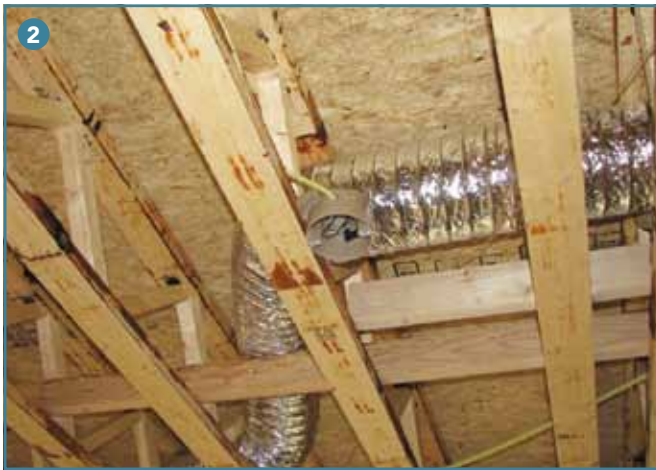
(2) Wood floor trusses like those in the 12 Washington Avenue structure.
