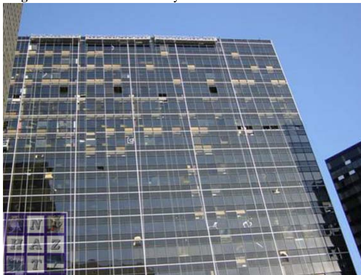
Figure 6 West face of 1250 Poydras.
