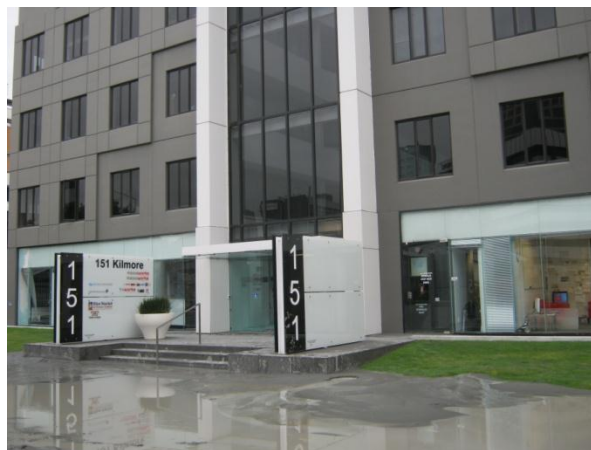
Figure 2.2. Evidence of liquefaction in Christchurch, New Zealand
