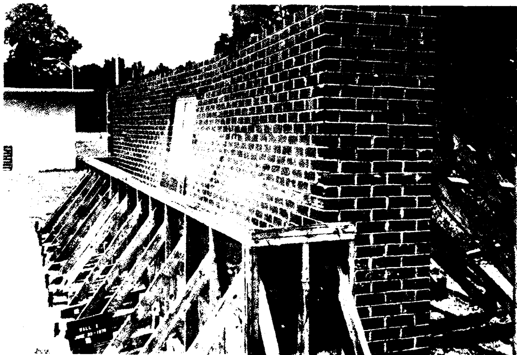
Figure 14. Wall 2. Wall failure, side view
