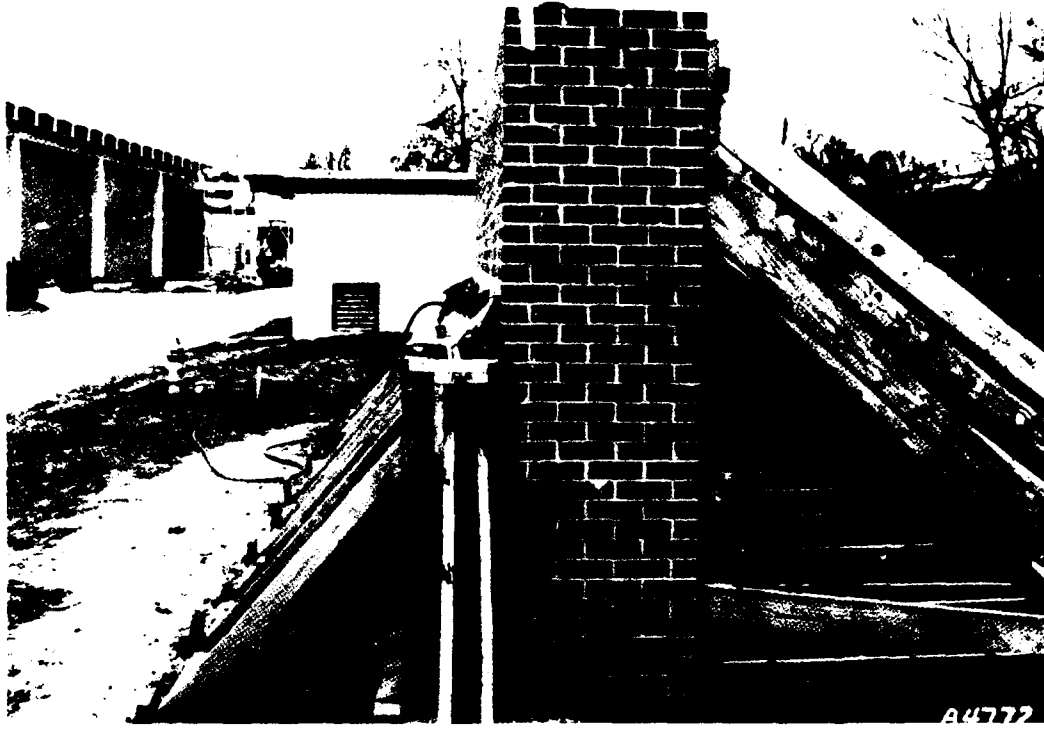
Figure 9. Wall 1. Wall deflection
