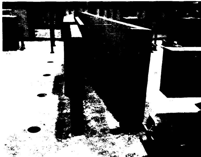
Figure 34. View 1. Bulkhead to contain water against the wall and closure
