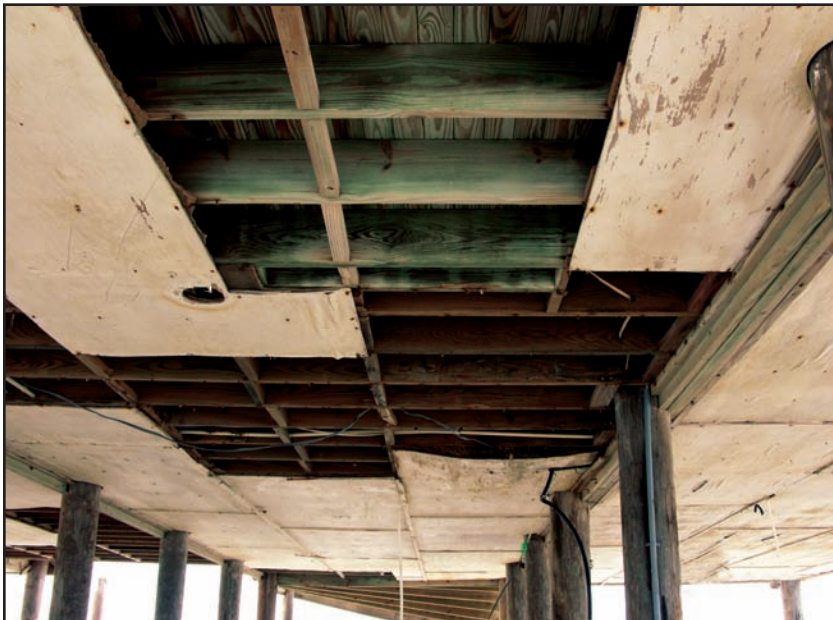
Figure 9-12. Example of an exterior floor covering system damaged by Hurricane Ivan. Note the good condition of the floor joists and flooring, due to their protection from salt spray prior to the storm. (Source: FEMA 489)
