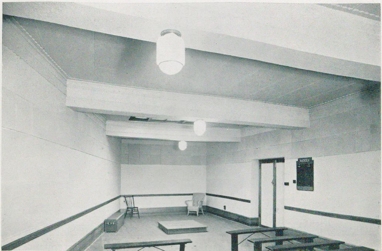
BAND ROOM, ROYAL MELBOURNE REGIMENT, VICTORIA STREET, MELBOURNE Ceiling and cornice lined with 1/2" Textured Donnacona.
