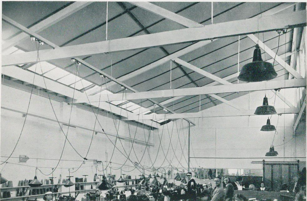
BELWORTH HOSIERY, 683 SYDNEY ROAD, COBURG, MELBOURNE Roof lining of \frac{1}{2} " Textured Donnacona.
