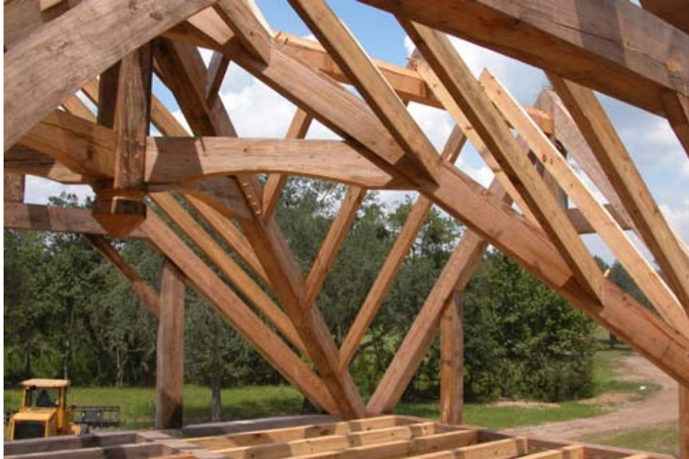
Unequal pitched joined timber frame valley system built using the Chappell Universal Square system. Main pitch 15/12, secondary pitch 9/12.
