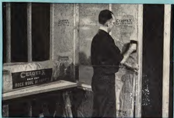
Pre-cut eight-foot lengths are ideal for rapid wall installation. Vapor-barrier with stapling flanges faces warm- or room-side.
