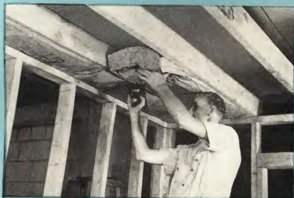
Stapler simplifies application, specially overhead. Self-spacing flanges permit easy application to joists, studs, rafters.
