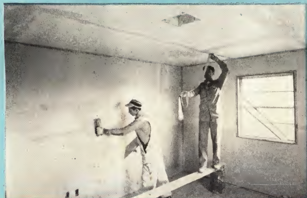
(B) This laminated construction is recommended for all ceiling and wall applications where greater rigidity plus insulation is desired.
