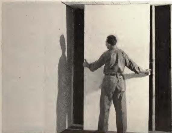
Lightweight Building Board is easily, quickly applied. Since the product comes pre-decorated, room occupancy can begin as soon as the last panel is installed.
