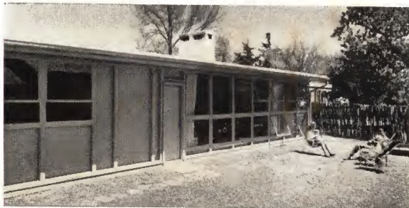
Large Cemesto Panels, extending from sill to top plate, provide single-thickness walls specially adapted to ranch-style design.
