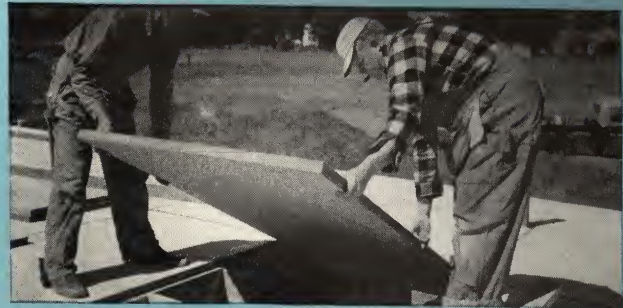
(A) Cemesto Panels are laid quickly and easily for roof decks.
