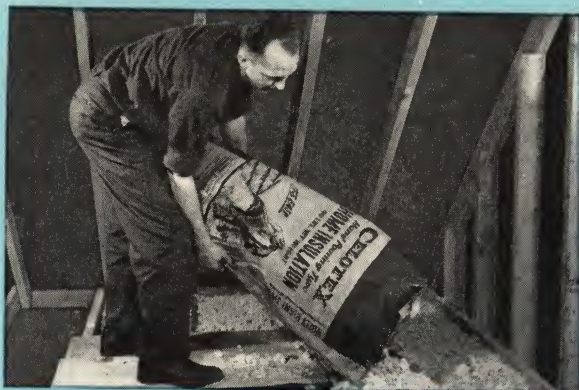
Hand-pouring type offers an easy method of insulating unfloored attic. Should be applied on vapor-barrier paper.
