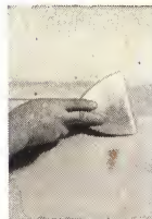
1. "Valley" formed by tapered edges is buttered with joint cement.
