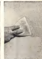
3. Two thin coats of joint finish are applied and feathered out about 12".
