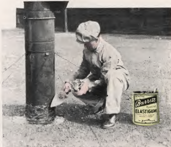
Junction of ventilator and roofing surface is made watertight and safe with Plastic Elastigum
