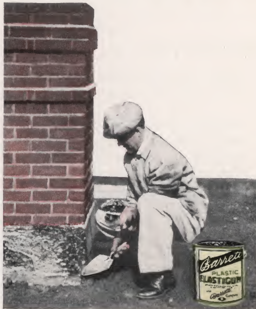
Plastic Elastigum makes weather-proof and leak-proof all flashing joints around chimneys and parapet walls
