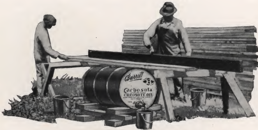
Brush treatment with Carbosota adds greatly to the life of lumber
