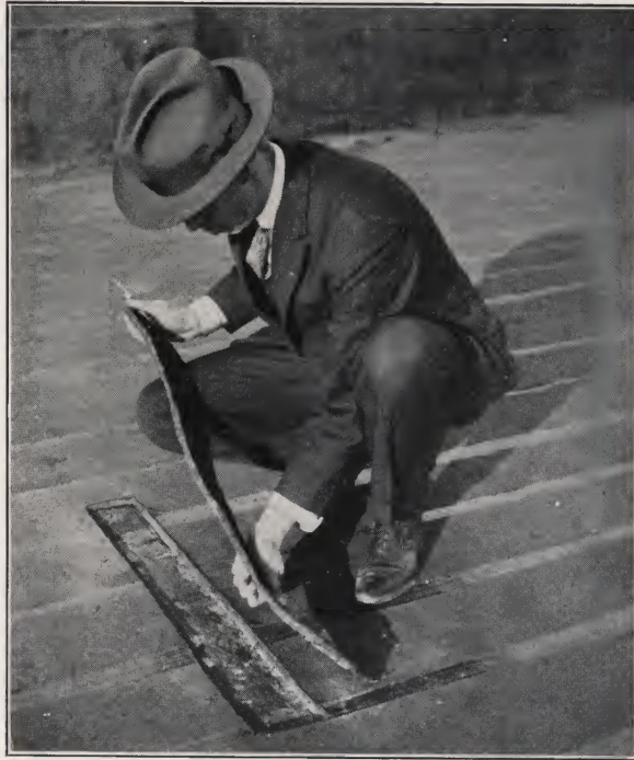
The famous "cut test" made by the Barrett Inspector before application of the slag or gravel surfacing
