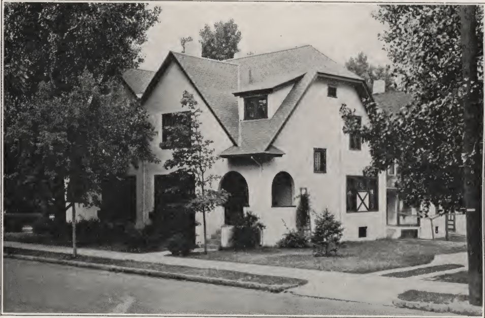
Residence at Springfield, Mass., re-roofed over old wooden shingles with Barrett Russet Brown Giant Shingles
