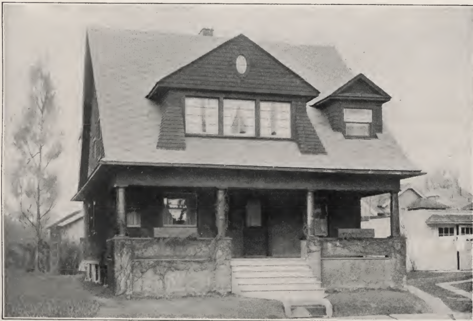
Residence at Toledo, Ohio, re-roofed over old wooden shingles with Barrett Wedgelock Shingles
