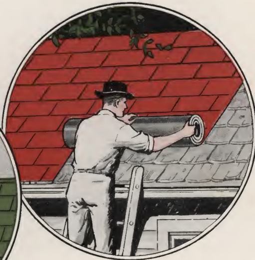
Style "V" is made especially for re-roofing over old wooden shingles
