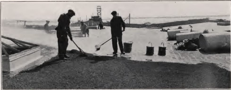
The poured top coat of a Barrett Specification Roof means just twice as much pitch on the surface as on an ordinary built-up roof
