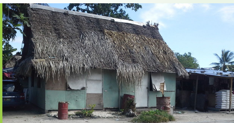
This typical residential dwelling on Tarawa, Kiribati may be built from asbestos cladding. However, testing would have to be undertaken to establish whether this is actually the case. Photo: PacWaste
