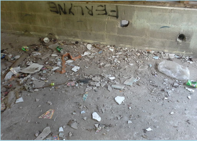
This vacant building in Nauru, littered with asbestos debris, appears to be frequented by young adults from the local community. Photo: PacWaste
