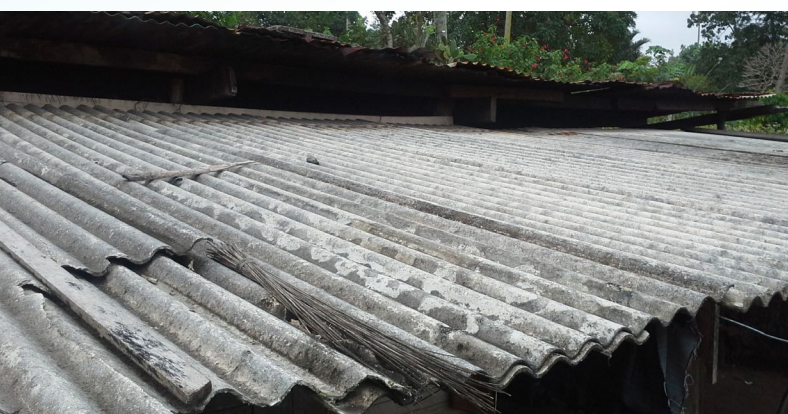
Corrugated asbestos cement roofing, pictured above on a building in Vanuatu, is relatively easy to recognise through visual inspection. Photo: PacWaste
