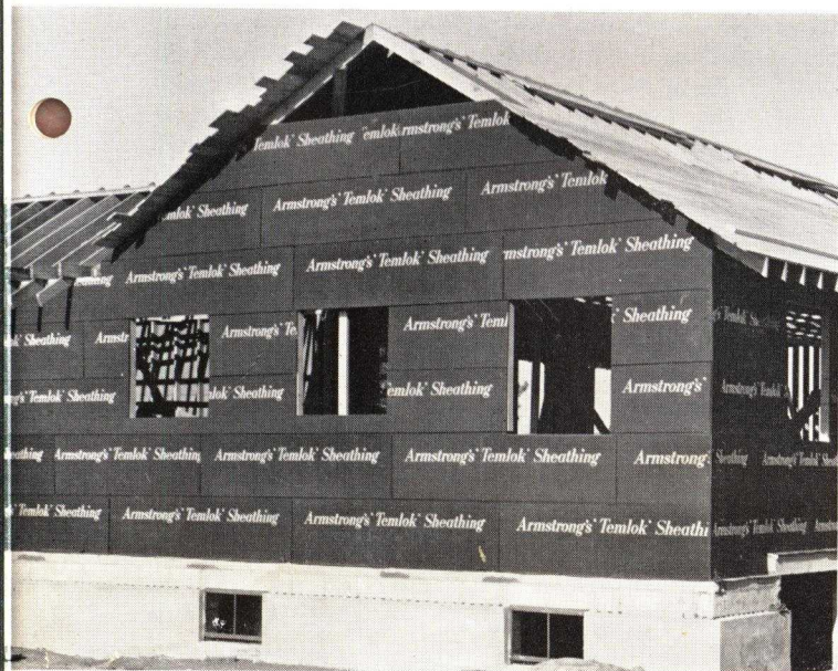
Temlok strengthens construction, goes up quickly and easily, and provides good insulation. Wood siding, brick, stone, or any other type of exterior finish can be used with this insulating sheathing.
