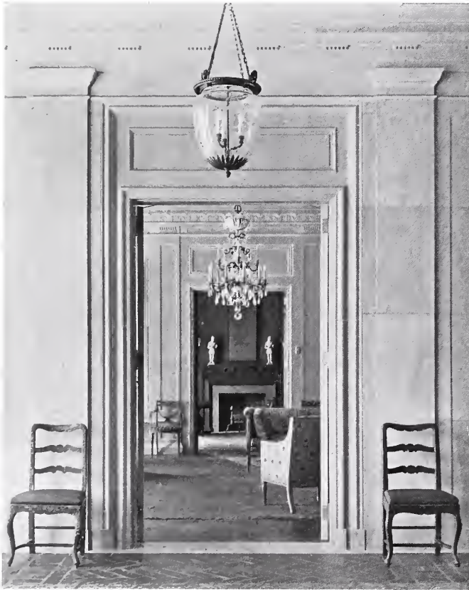
Hall Doorway to Morning Room
