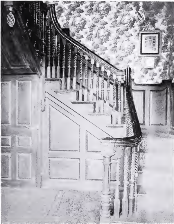
Stairway in the Hannah Robinson House
