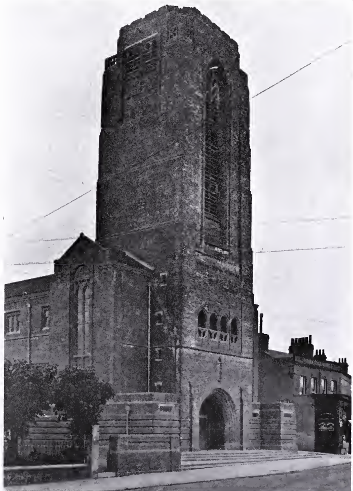
Tower on West End, Catholic Church, Northfleet, Kent
