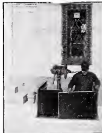
Doors opened and automatically locked. Operator ascending iron ladder to sidewalk.
