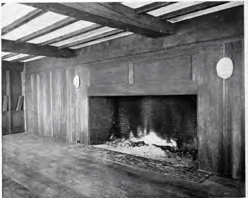
Detail of Restoration Work, Old House at Bolton, Mass. Biglow & Wadsworth, Architects
