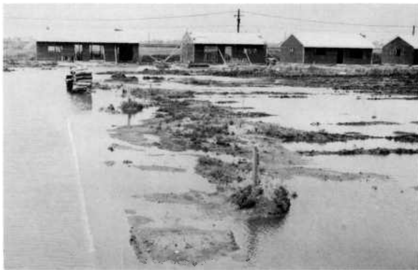
The poorly drained soil on which these houses are being built will not be satisfactory for septic-tank filter fields.
