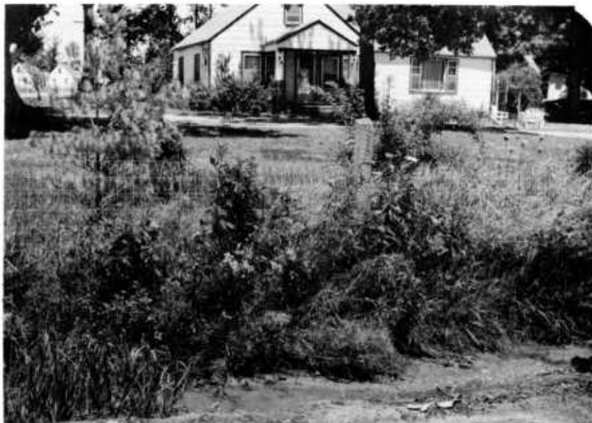
The septic tank and filter field for the suburban home (background) is located just beyond the wire fence (foreground). The soil is Iredell silt loam, which has a very plastic clay subsoil that is almost impermeable when wet. The roadside ditch in the immediate foreground is filled with septic-tank effluent that has seeped from the filter field, even though this picture was taken during a summer drought.
