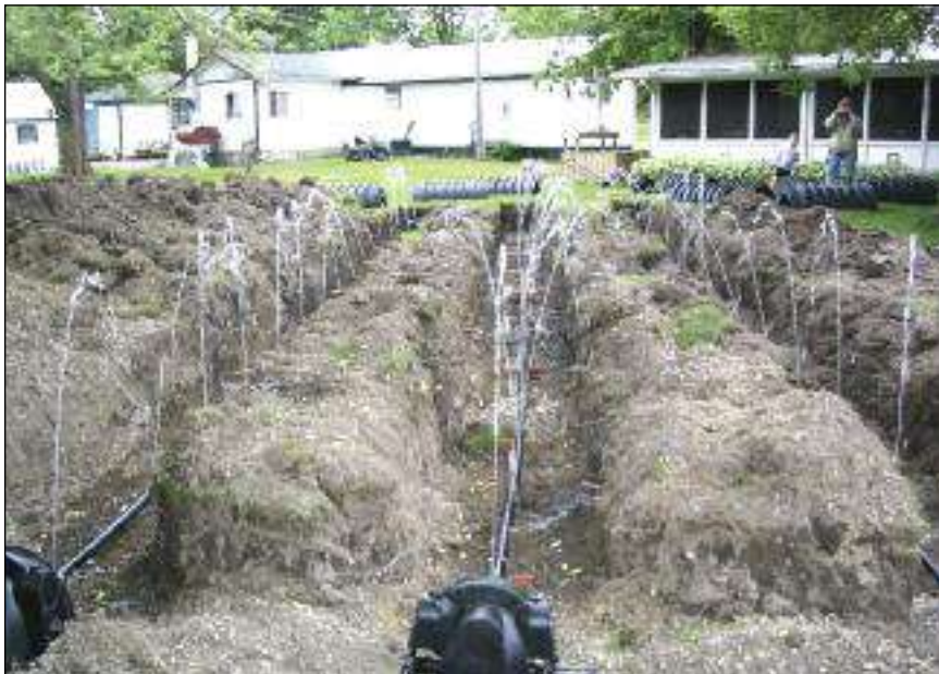
Shallow buried trenches showing equal distribution methods. Note: before placement of chambers.
