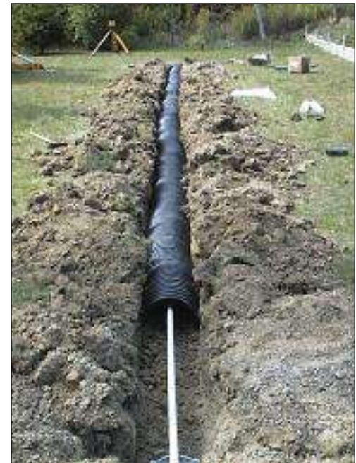
Single line shallow buried trench.
