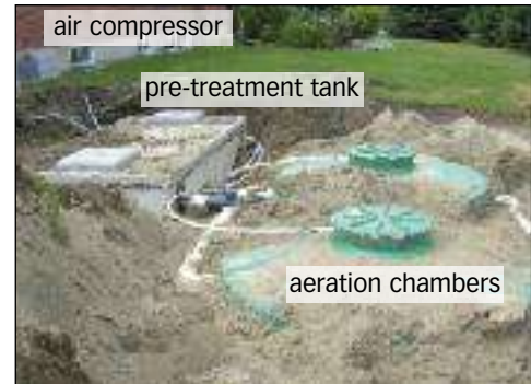
Large sewage design flows may require more than one aeration chamber.
