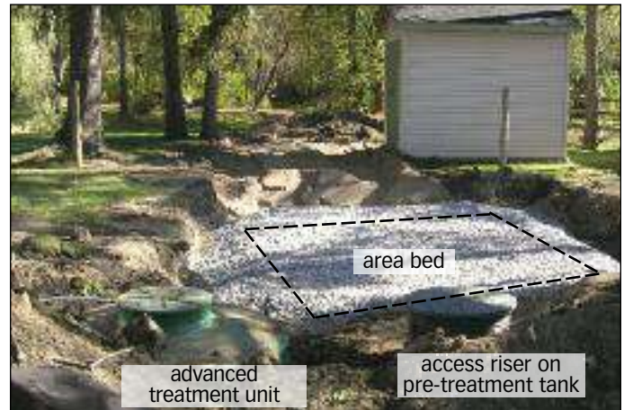
An area bed in a small space.
