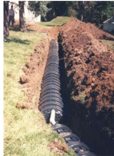
Underground leaching chamber installation on an onsite wastewater system. Photo: State Conservation Service Kansas
