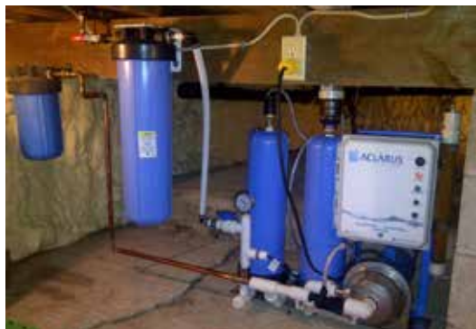
A domestic Aclarus unit installed in a household handling a flow of 3000 L/day
