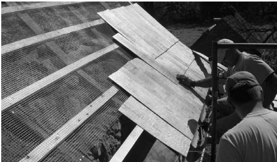
Fig. 7. The Saal, Ephrata Cloister, 2004. The roofers are installing a double starter course of side-lap shingles, with the bottom layer slightly shortened. This shortened course and the kick in the eave make it easier to keep the tips of the shingles down in the first three courses. The \frac{1}{2} -inch hardware cloth is used here as a squirrel barrier.
