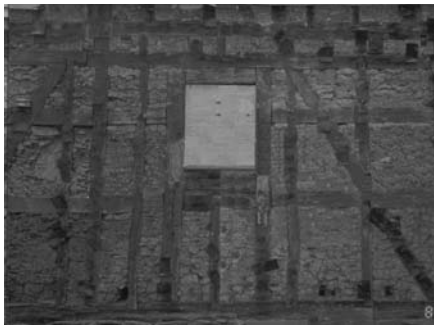
Fig. 2. The north gable end of the Saal at Ephrata Cloister during a siding-restoration project in 1998. This image shows typical eighteenth-century fachwerk, or half-timbering, with limestone and clay nogging. The scaffold has been edited out of the digital scan.
