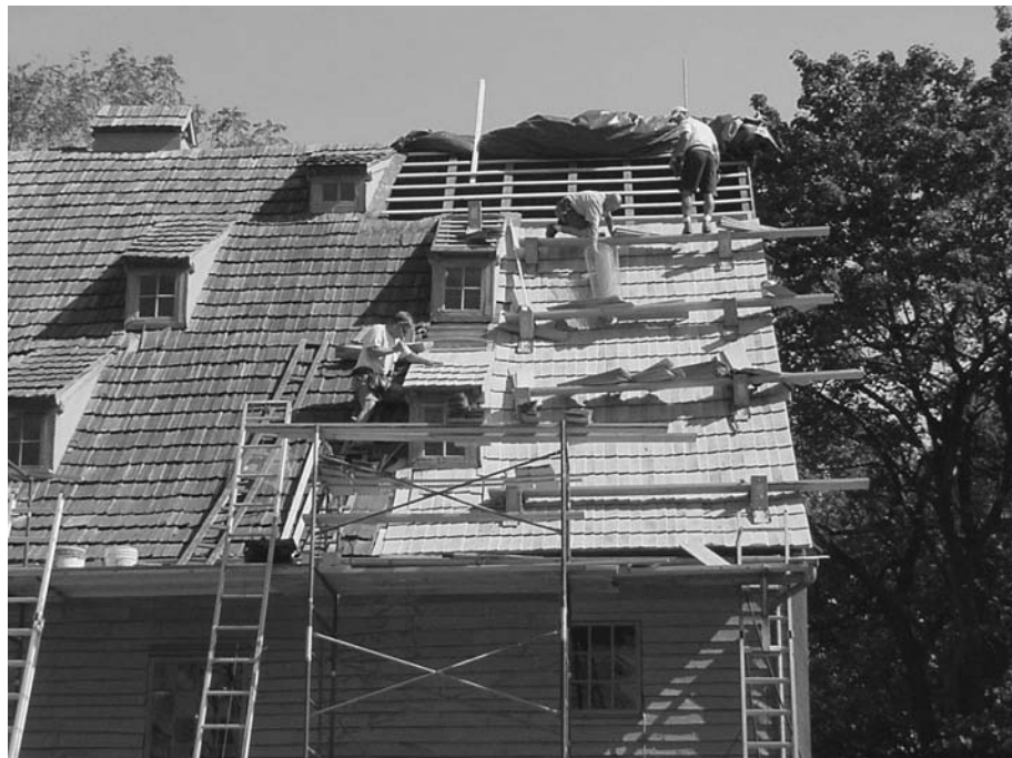
Fig. 1. The layout of side-lap shingles makes it relatively easy to work to a vertical edge. Nineteen-year-old western red cedar shingles are being replaced with handmade red oak shingles at the Saal, or meetinghouse, at Ephrata Cloister. Because the courses of side-lap shingles are not staggered, the roofers are able to work to a straight, vertical edge from the eave to the ridge of the roof, making it much easier to tear off and replace roofing on buildings of this size. All images by the authors.
