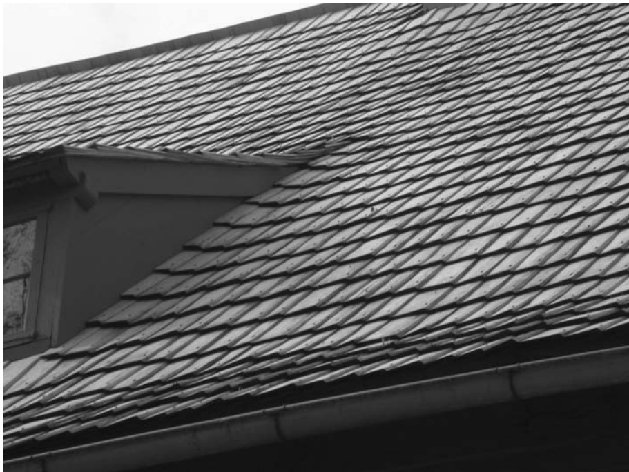
Fig. 9. The Saron, Ephrata Cloister, 2005. Each row, running vertically, contains shingles of like width. Courses run horizontally. Also visible are the kick at the eave and the upward flare of the roof at the side of the dormer created by a tapered fillet board. There is no metal flashing.
