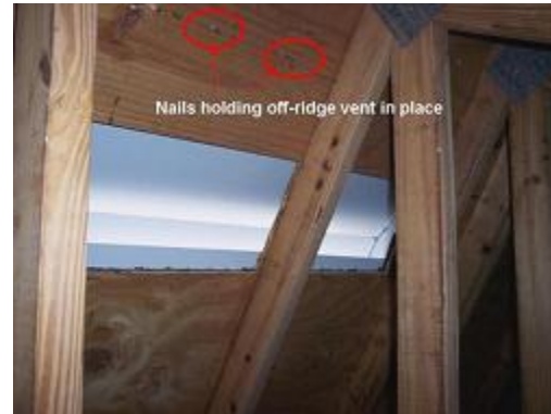
Off-ridge vent viewed from inside attic. Note the nails used to attach the vent to the roof deck (click image for larger version)
