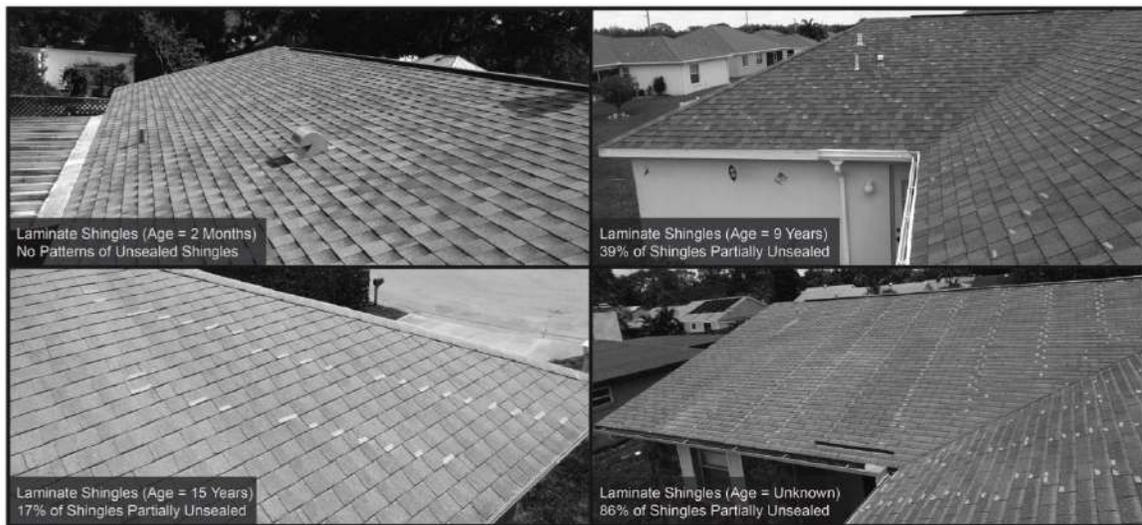
Figure 4-3. Location of partially/fully unsealed three-tab and laminate shingles (tape marks).
