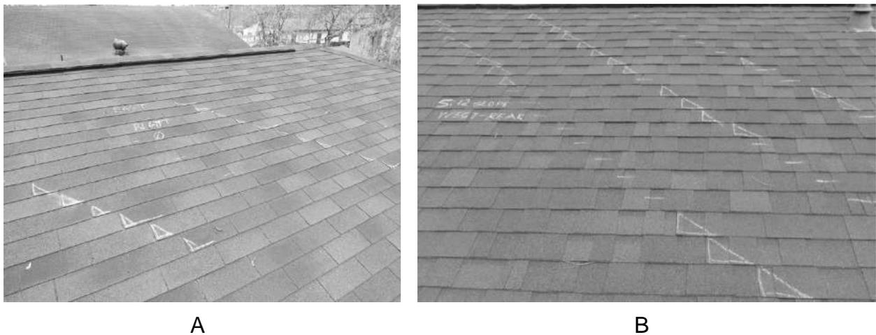
Figure 4-4. Shingle roofs located in Houston, TX with partially unsealed shingles located by triangular chalk marks and fully sealed shingles located by dash marks. A) Three-tab shingles and B) laminate shingles.
