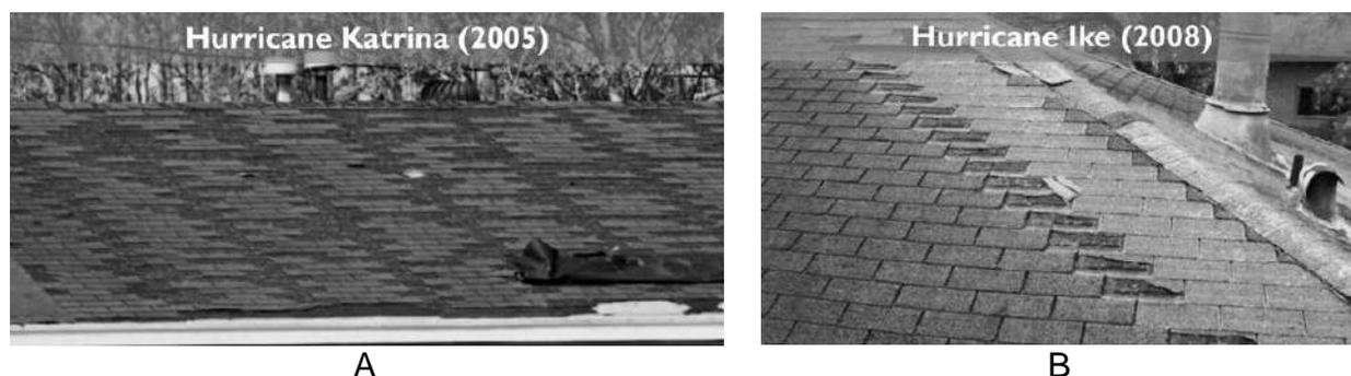
Figure 4-7. Blown off three-tab asphalt shingles. A) Hurricane Katrina in 2005 and B) Hurricane Ike in 2008.
