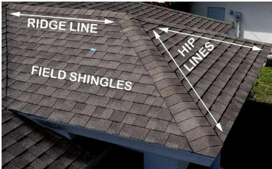
Figure 2-1. Asphalt shingles are installed in the field of the roof with additional shingles along hip and ridge lines.
