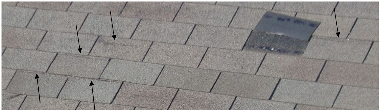
Numerous creased shingles (highlighted with arrows) indicate that they've flapped back and forth repetitively in the wind, probably over a long period of time. Eventually these shingles will tear and blow away, even under mild winds not associated with severe weather.
