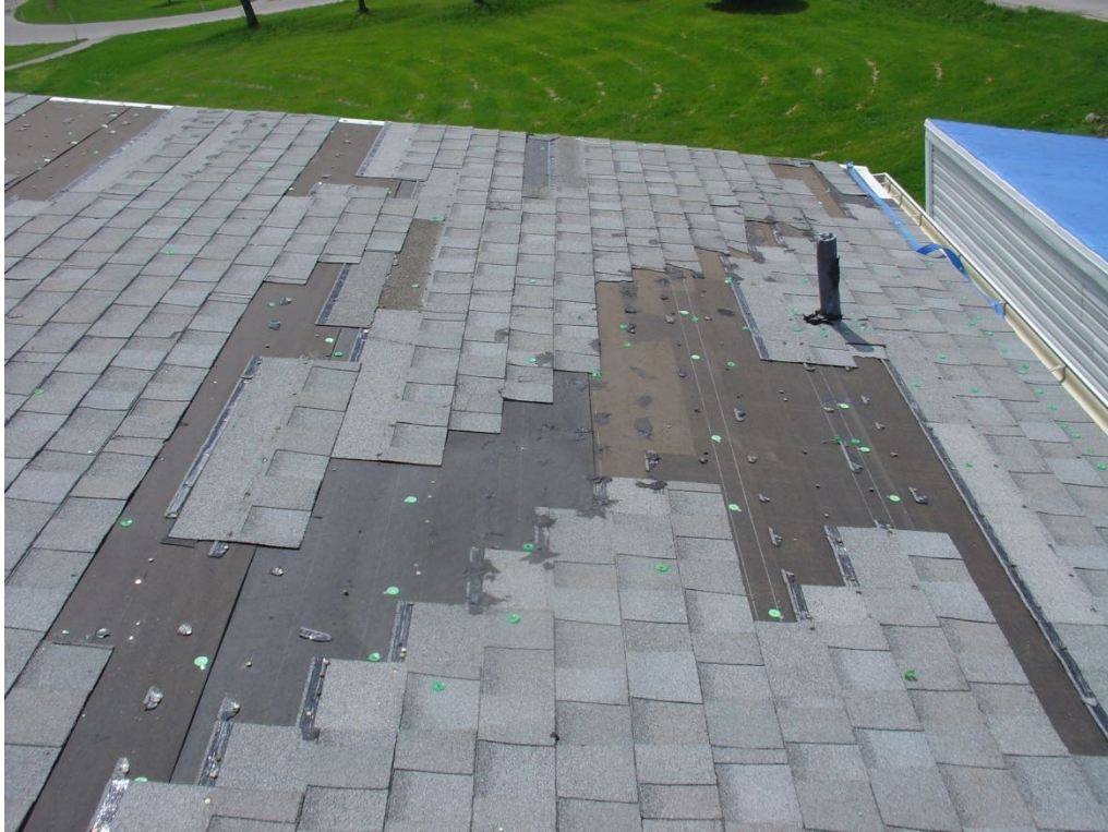
A poorly-sealed dimensional shingle roof that encountered strong, but not severe, wind.
