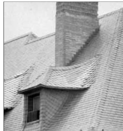
Because of the roof's visibility, the slate detailing around the dormers is important to the character of this structure. Photo: NPS files.
