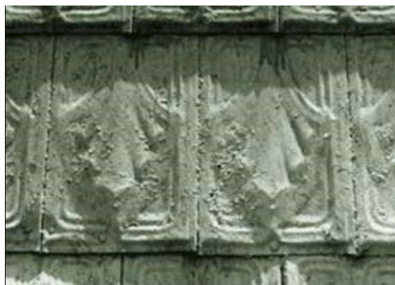
Tin shingles, commonly embossed to imitate wood or tile, or with a decorative design, were popular as an inexpensive, textured roofing material. Photo: NPS files.
