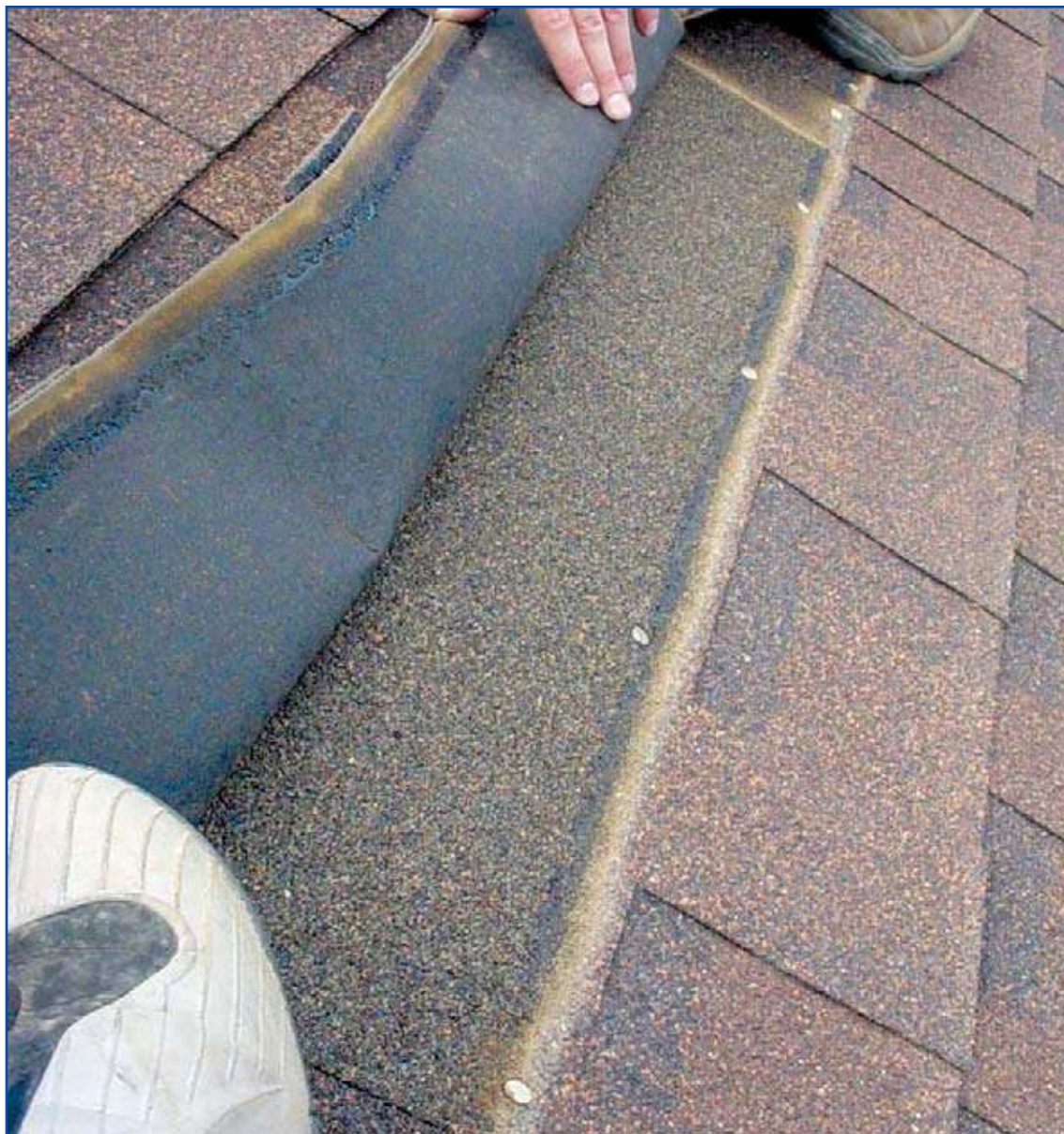
Photo 3: The nails are placed not only in the wrong locations, but also above the asphalt seal line, resulting in penetration of only one of the laminate shingle layers.
