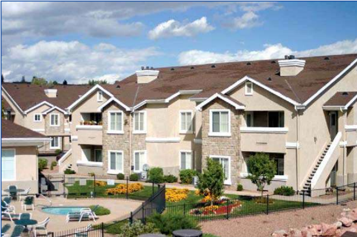
Photo 1. Overview of a building on the property, showing the loss of shingles.
