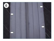
ii. Ribbed Valley Metals that have a crimped edge or an outside turn back may be fastened using metal clips/ cleats. Metal clips/cleats engage the crimped edge or outside turn back and are fastened to the roof deck. (Figure 7)
