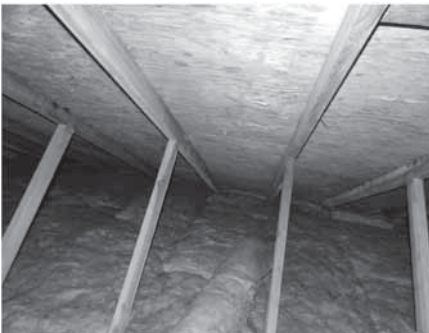
Notice how mold is starting to grow on the underside of the roof deck
