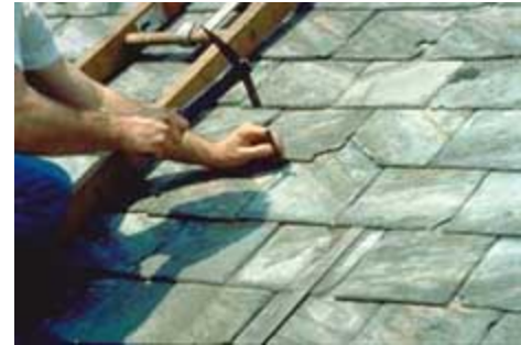
Slate roof repair. Photo: Jeffrey S. Levine.
