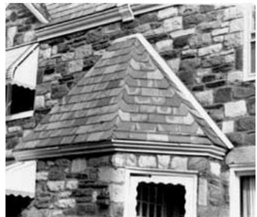
The white blotches on these Pennsylvania Soft-Vein slates indicate areas where gypsum is leaching out onto the surfaces of the slates. Photo: Jeffrey S. Levine.
