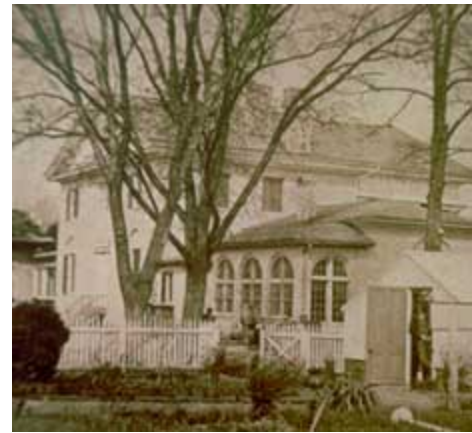
Prior to replacing a roof, historical documentation is gathered (such as photo documentation) to determine the roof configuration. Photo: NPS files.
