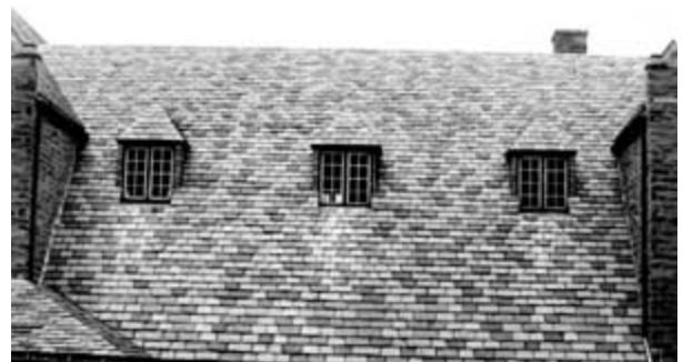
This graduated slate roof is composed of large, thick slates at the eave which are reduced in size and thickness as the slating progresses to the ridge. Photo: Jeffrey S. Levine.
