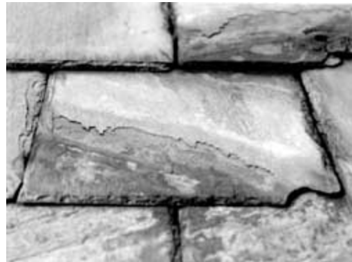
Paper thin lamination can be seen flaking off this weathered, 120 year piece of Pennsylvania Hard-Vein slate. Photo: Jeffrey S. Levine.
