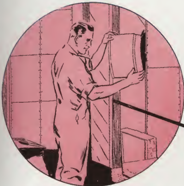
Flintkote Rock Wool Bats fill hollow walls and attic spaces to a uniform thickness and density.
