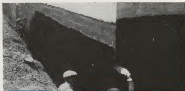
This exterior concrete wall below grade is protected against water and moisture infiltration by applying Flintkote Static Protective Coating.
