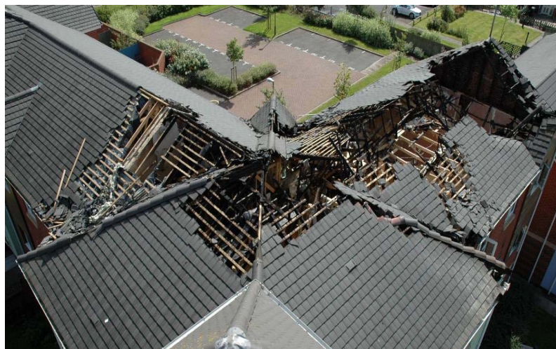
Figure 8 – Aerial view showing damage to roof structure
