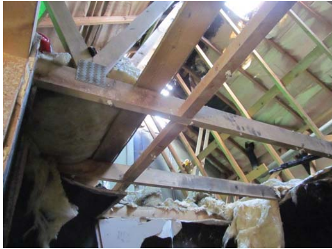
Figure 10 – Undamaged roof trusses above seat of fire
