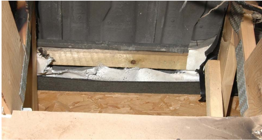
Figure 4 – Combustible membrane under roof covering
