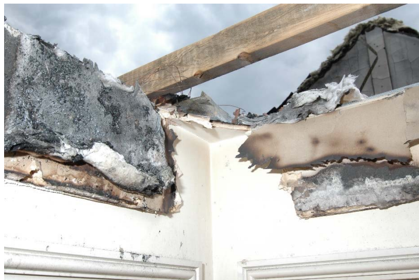
Figure 3 – Mineral wool fire-stopping along pitch of roof in the background of the photograph
