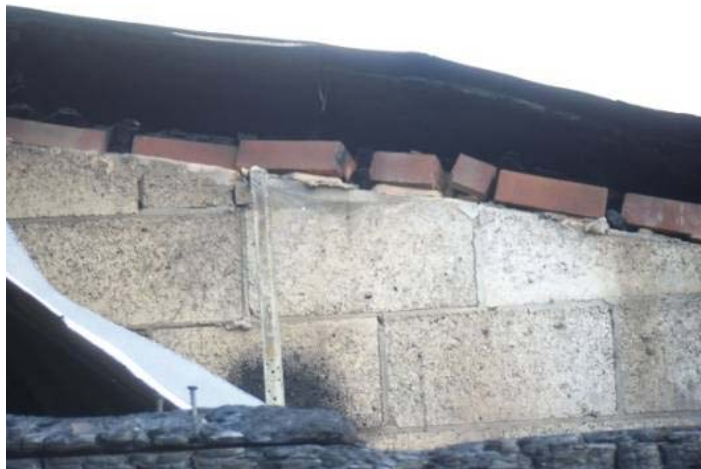
Figure 6 – Attempt to follow roof profile over compartment wall
