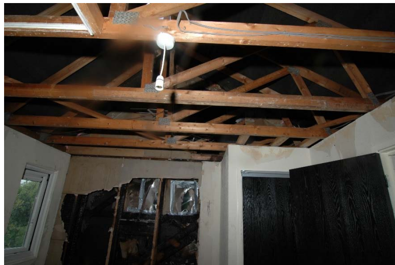
Figure 11 – Top floor of property showing fire damage in party wall but roof trusses are unaffected by the fire due to compartmentation
