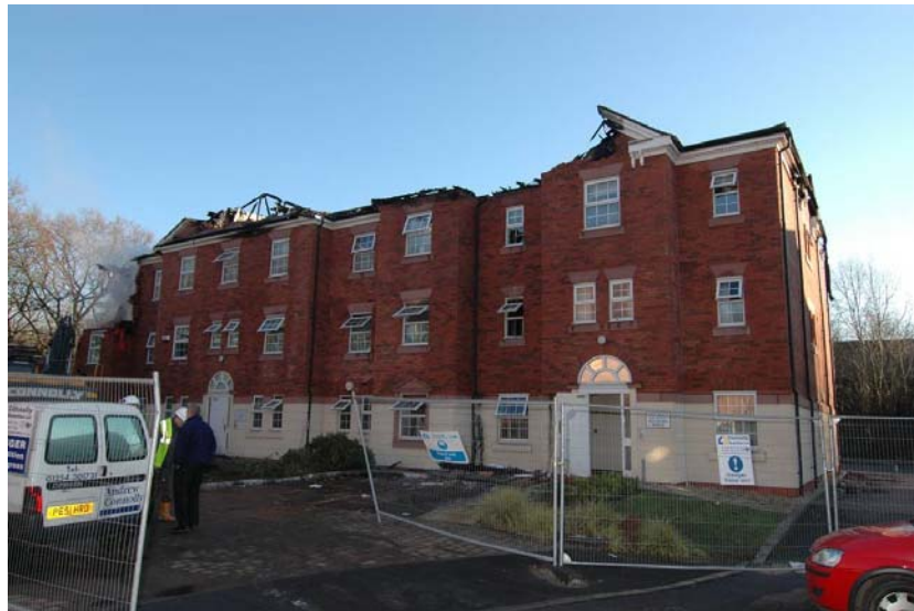
Figure 2 – Block of flats showing the area of fire origin and damage to roof level. Arrow A indicates point of fire origin. Arrow B indicates point of break out at roof level
