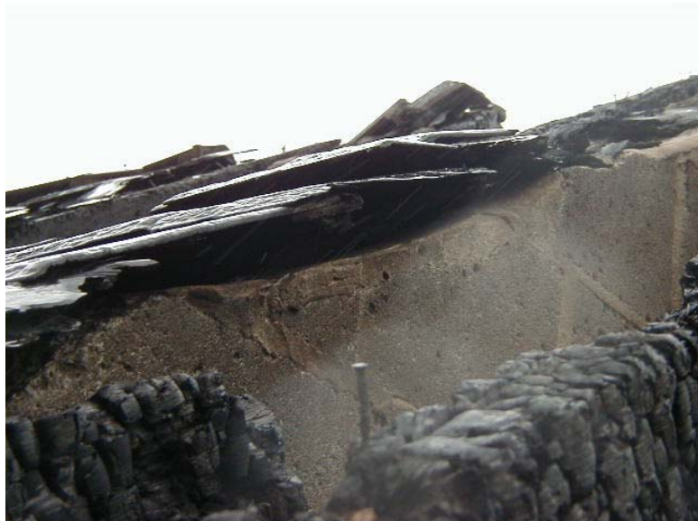
Figure 1 – Lack of fire stopping between compartment wall and roof covering
