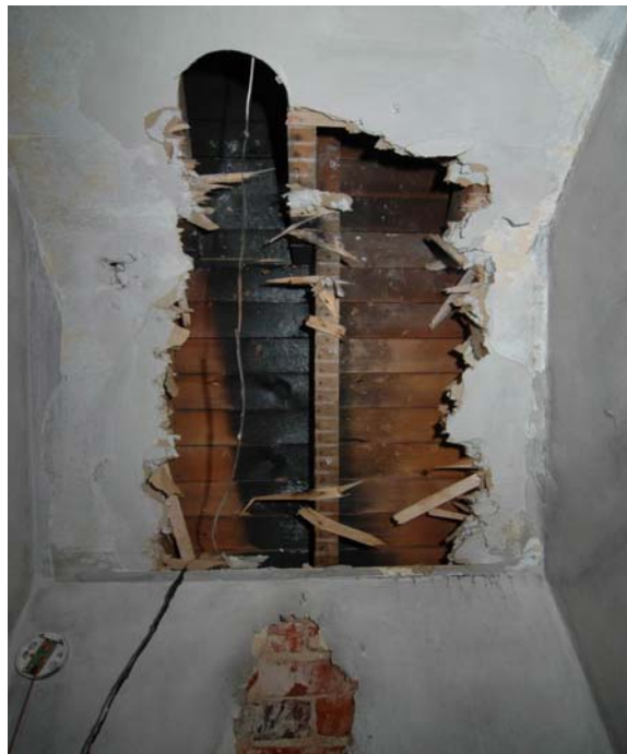
Figure 9 – Close up of fire damage to pitch roof (arrow showing direction of fire spread from wall cavity)
