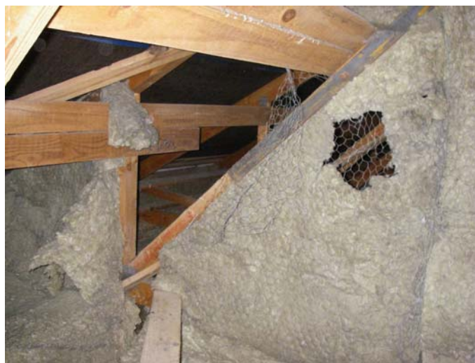
Figure 5 – Fire stopping in poor condition (Image courtesy of London Fire Brigade)
