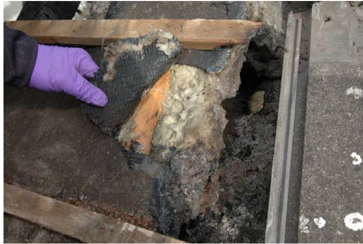
Figure 7- Fire stopping against underside of sarking felt but not pushed up against underside of roof tiles
