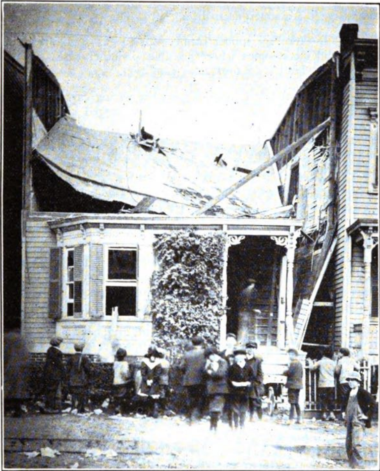
Wreck of a house due to hunting a leak of illuminating gas in the second story with a lamp. Comment is unnecessary.
