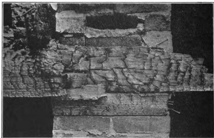
Chimney one brick thick unlined. Floor construction built into chimney wall. Floor timbers also in contact with it. Vibration loosened brick and caused fire.
