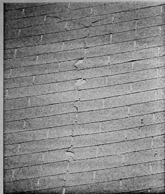
Figure 2. Fiberglass shingles that fail early usually crack, either vertically up the roof over many courses of shingles, or horizontally and diagonally across tabs.
