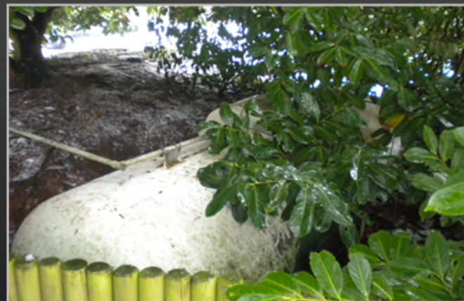
Tank in overgrowth
